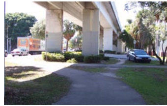
Missing trail segments
