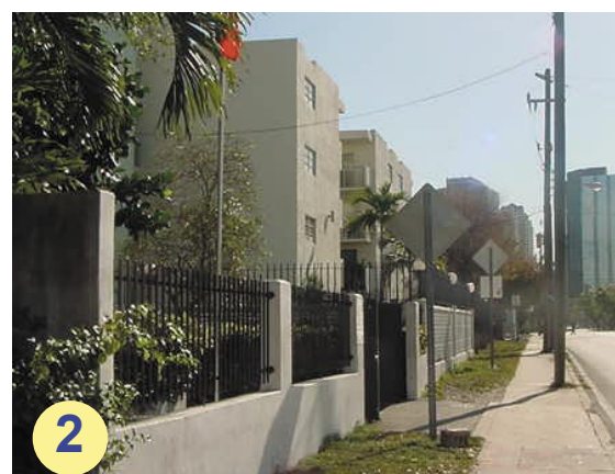
Facing east along the north side of SW 13th Street. Buildings along this Zone relate poorly to the public realm on both sides of the street. Here a six foot wall visually and physically separates the building from the street reducing the quality of the urban experience in this area.
