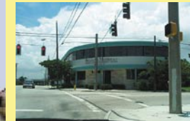
NW corner of SW 2nd Ave and SW13th St (Zone 1)
