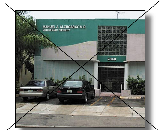
Front loaded parking - backing into the street shall be prohibited
