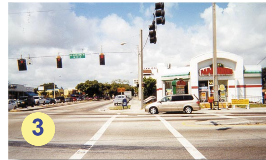
Corner of SW 22nd Ave. Wide crossing distances and poor aesthetics are typical conditions found at the major intersections throughout the corridor. Opportunities exist to beautify these elements by introducing different materials such as colored concrete crosswalks and reducing crosswalk widths wherever possible.
