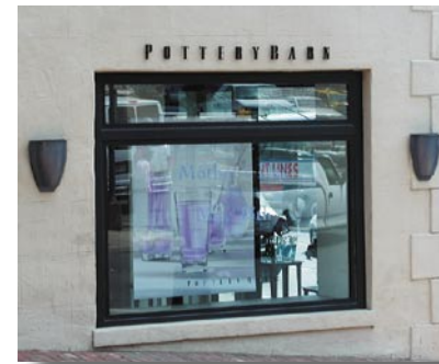
Window with concrete trim
