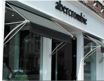
Canvas awning supported by metal internal structure
