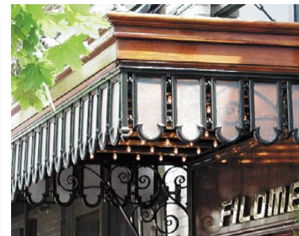
Wood and glass canopy supported by metal hangers
