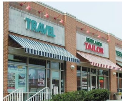
Brick walled building
