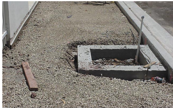
Step 1 - Laying the structural soil underneath the sidewalk and compacting it.
