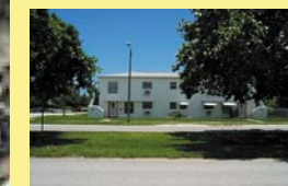
Typical residential building (Zone 2)
