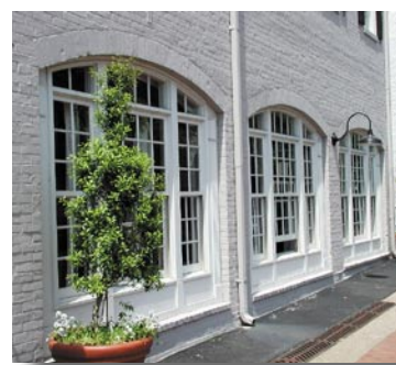
Windows with brick trim
