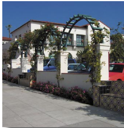
Trellis, low wall and benches shielding parking
