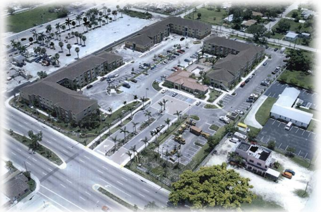
The Corinthian completed - June 8, 2007
