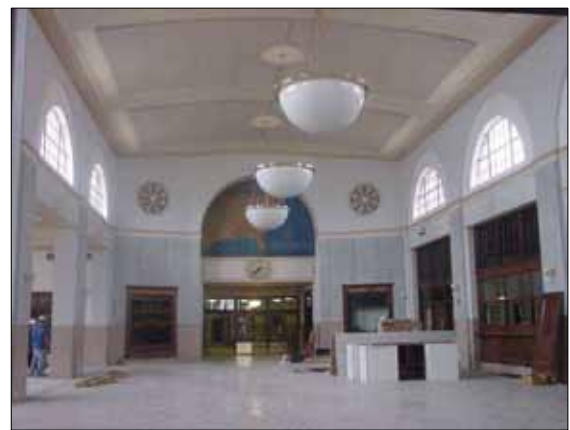
(i) Depot building during rehabilitation to serve as rail station
