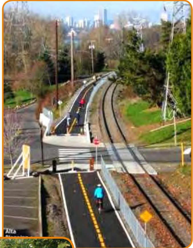
Springwater Corridor Trail, Portland, Oregon
