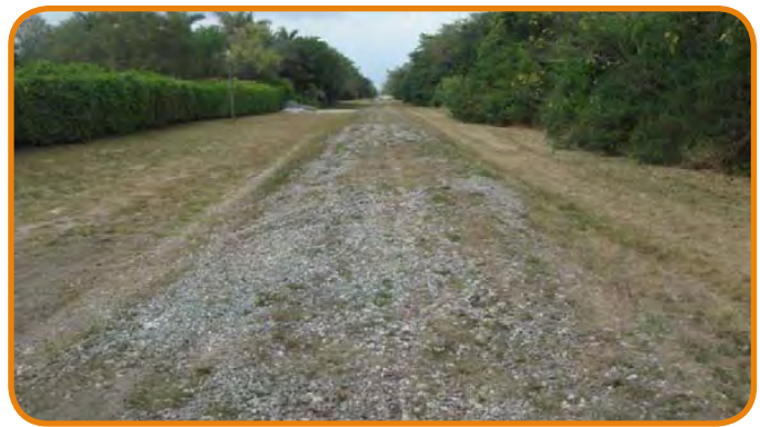
Railroad tracks have been removed south of SW 12th Street
