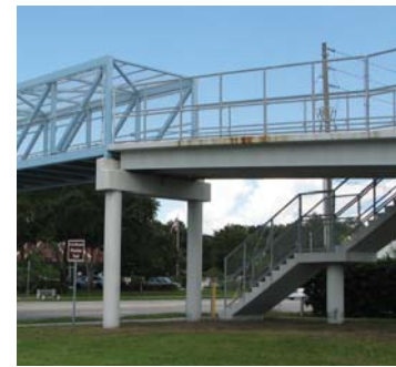
Ramp approach to bridge with stairs
