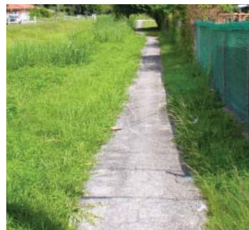
Safe Route to School sidewalk near SW 22nd St.
