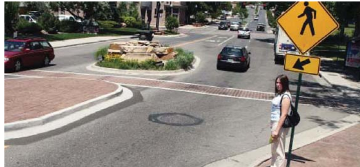
Example of improper use of a chicane to slow motorist with adjacent bus bay leading to unsafe crossings
