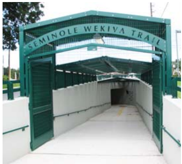
Hwy 434 tunnel entrance ramp and gate
