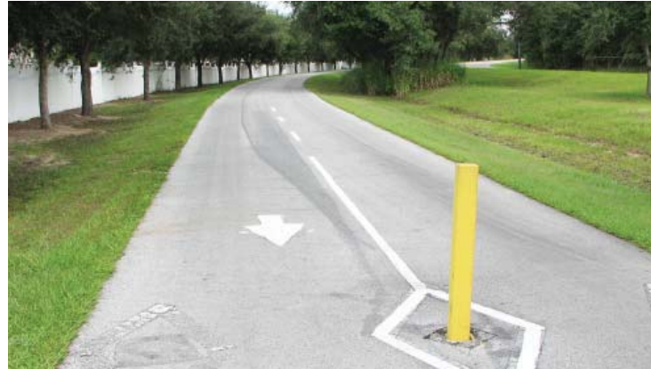
Single center bollard used at each at-grade crossing approach
