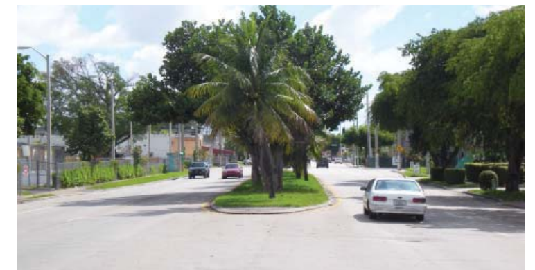
SW 24th St. existing roadway view with landscaped median without pedestrian refuge island
