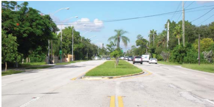
SW 72nd St. existing roadway condition with landscaped median and lack of pedestrian refuge island
