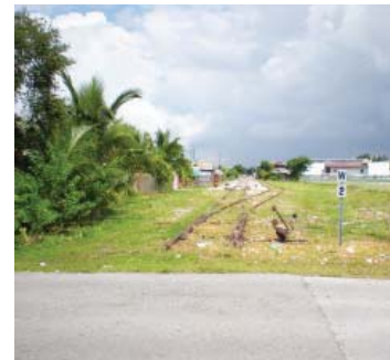
SW 12th St. end of existing railroad tracks
