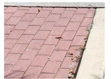
Example of concrete pavers
