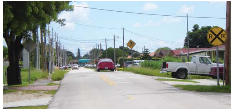
SW 21st St. existing corridor condition with railroad crossing striping and signage
