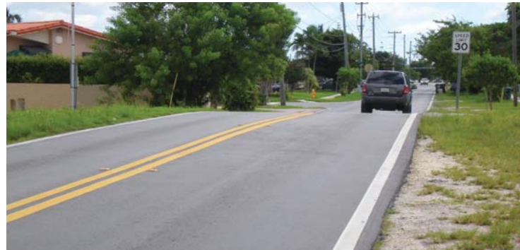
SW 16th St. local street crossing with high speed
