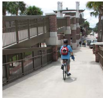
ADA accessible ramps for Above-Grade crossing
