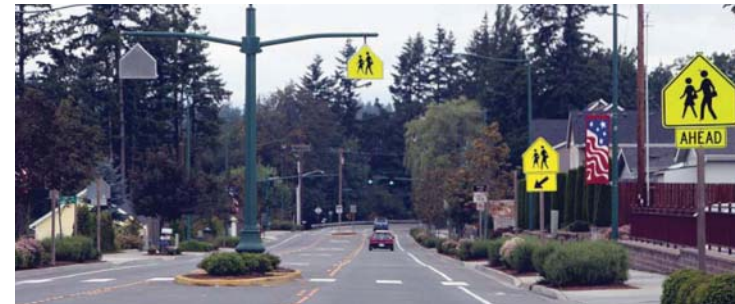
Example of sign redundancy with overhead signs and roadside signs
