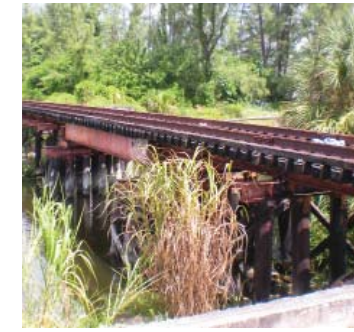
Tamiami C-4 Canal Bridge
