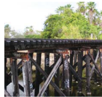
Coral Gables C-3 Canal Bridge
