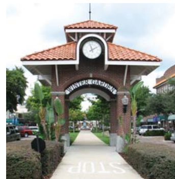
Pavilion with signage forms a grand gateway feature
