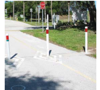
Bollards at controlled entrances
