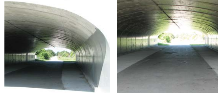
Below-grade crossing typical tunnel with 25-30' width and 15'+ height
