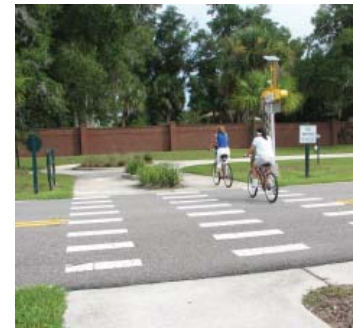
Typical Seminole crossing markings
