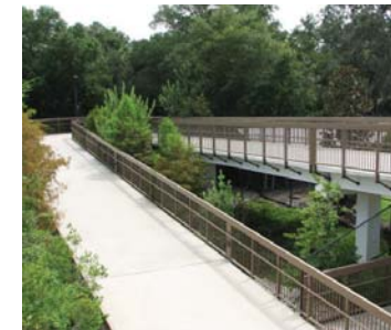
ADA accessible ramp to pedestrian bridge
