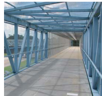
'Caged' bridge structure
