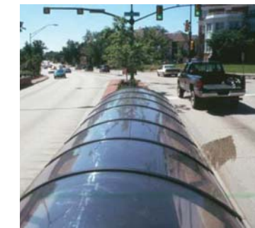
Example of a tunnel skylight located in a roadway median
