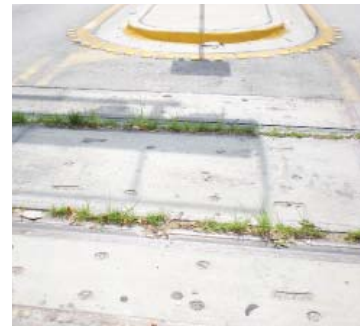
West Flagler St. existing tracks
