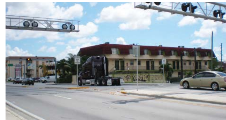
West Flagler Street existing railroad crossing with nearby signaled intersection
