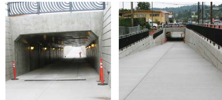
Below-grade crossing at 68th Ave. NE with wide tunnel width
