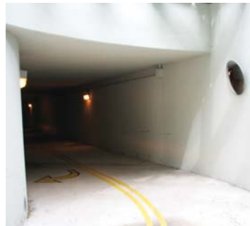
Hwy 434 tunnel entrance
