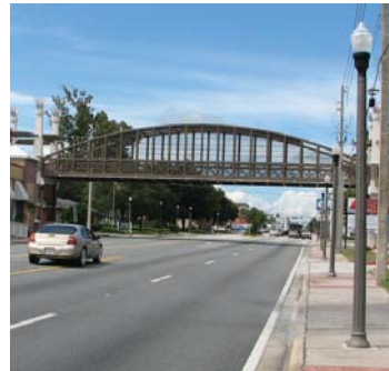
Above-Grade crossing in Apopka, Florida
