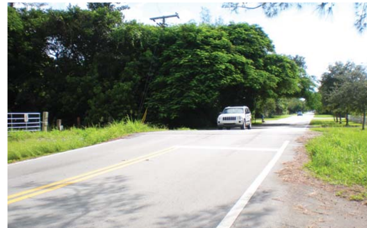
SW 64th St. local street crossing with high speed
