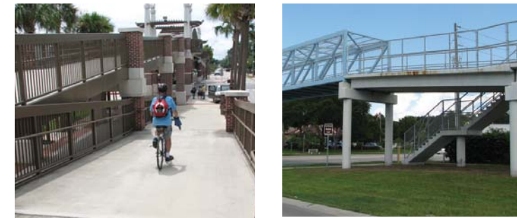
Above-Grade crossing in Apopka, Florida
