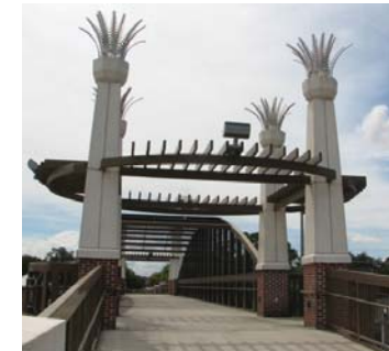
Iconic bridge along West Orange Trail
