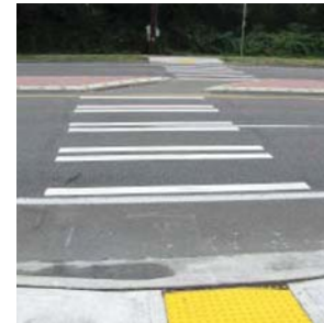
Enhanced crosswalk markings
