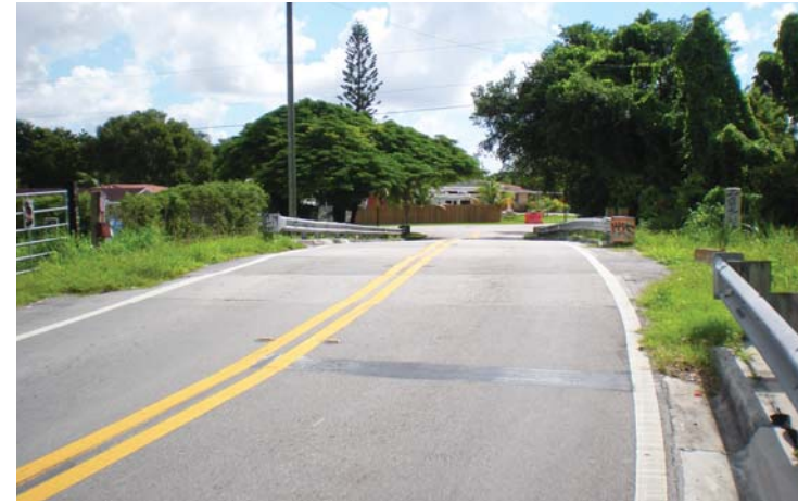
North Waterway Drive with no sidewalk access
