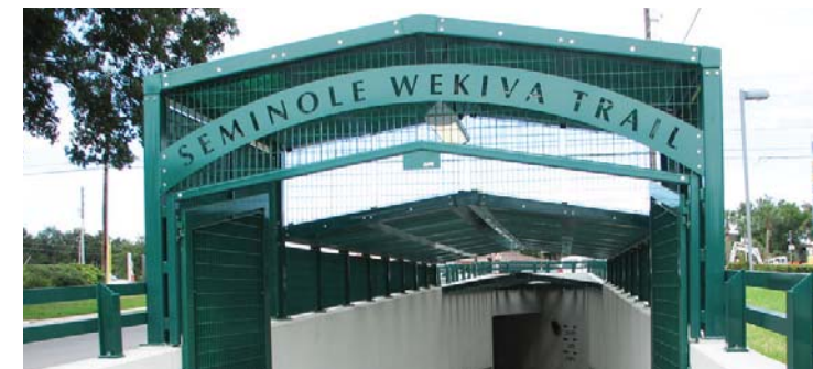
Seminole Wekiva Trail Below-Grade crossing tunnel entrance
