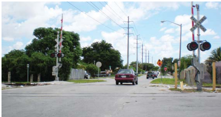
SW 4th St. existing railroad crossing
