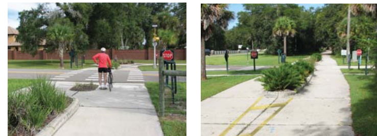
Seminole-Wekiva Trail crossing with raised median and divided crossing approach
