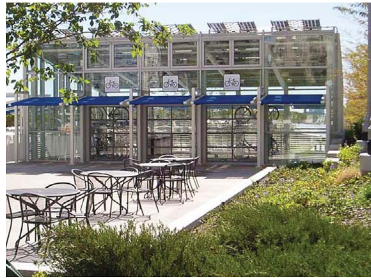
McDonald's Cycle Center (bike hub) facility with outdoor seating www.nycc.org
