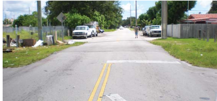
SW 12th St. existing local street crossing
