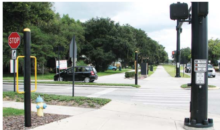
At-Grade crossing with push button crosswalk signal and minimum refuge island
