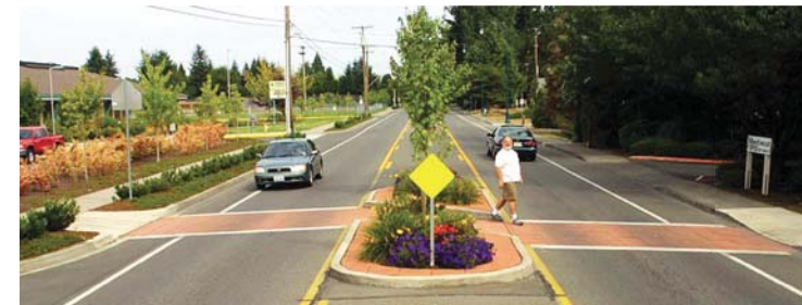
Proper geometrics for a non-arterial crosswalk with an angled pedestrian refuge island
