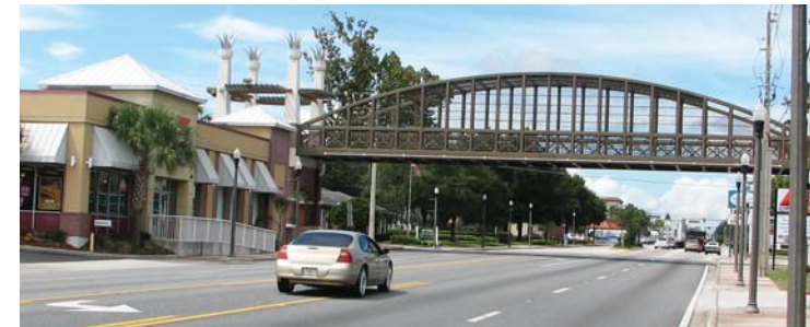
Example of an above-grade trail crossing along the West Orange Trail, Orlando Florida
