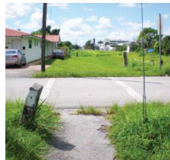
Existing crosswalk with signage
