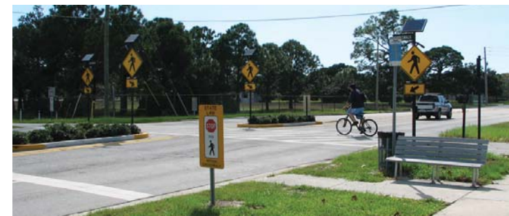
Highly marked mid-block crossing with stutter signals (flashing beacons) and bus stop
