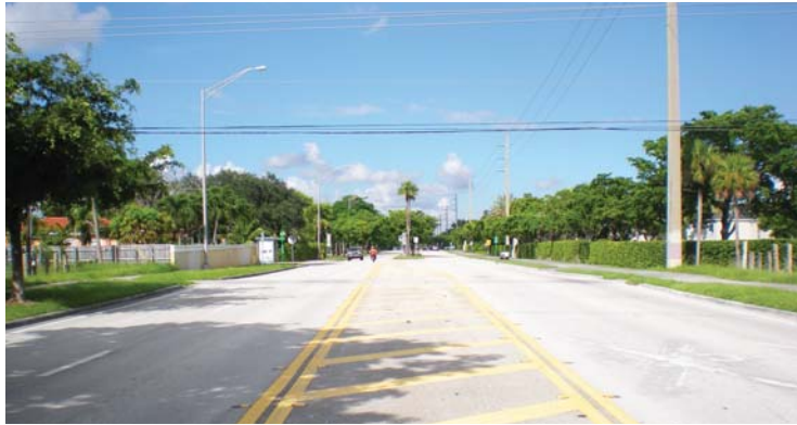
SW 56th St. existing corridor condition with no pedestrian refuge
