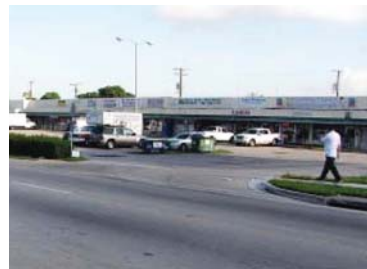
The above images show a poor example of driveway access management which encourages high speeds turns and poorly defines crosswalk area
