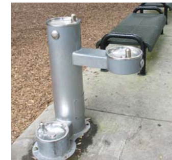
Example of ADA accessible drinking fountain
