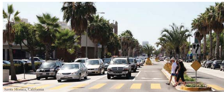
Santa Monica, California Example of refuge island and crosswalk markings for an arterial crossing
