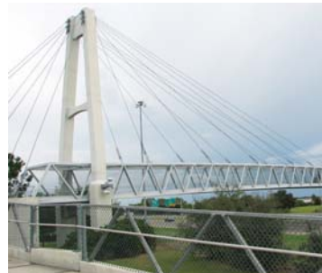
I-4 ADA compliant bridge
