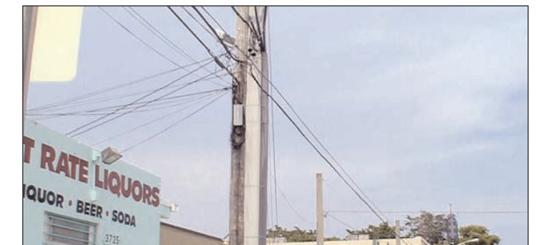
Above: Existing overhead wires and utility poles
