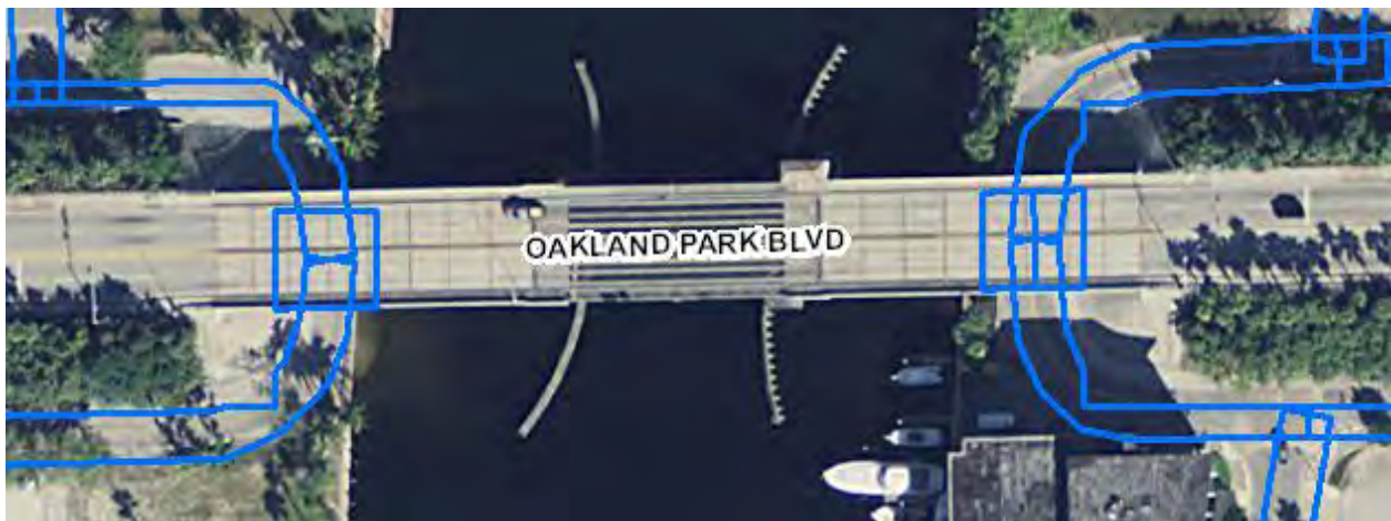
Figure 18: This bridge crosses the Intracoastal Waterway. It appears to have nearby inundation, but the blue, flooded streets shown are actually U-shaped streets under the elevated bridge and do not affect its function.
