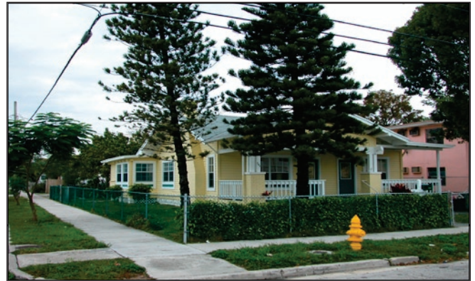
A recently restored wood frame house in East Little Havana
