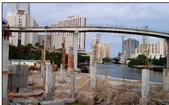
One Riverview Square under construction (2)
