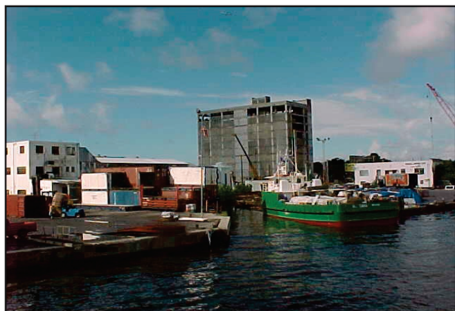
Brickell Shipyards- An adaptive reuse/redevelopment opportunity (8)
