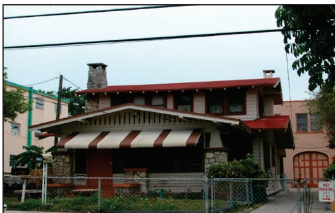
A wood frame house with coral rock piers in East Little Havana
