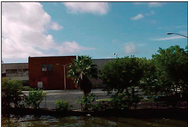
Redevelopment site- The former Miami News Site (20)
