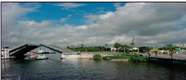
5th Street Bridge (18)
