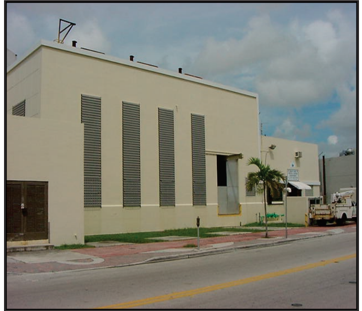
Pump Station No. 1 today
