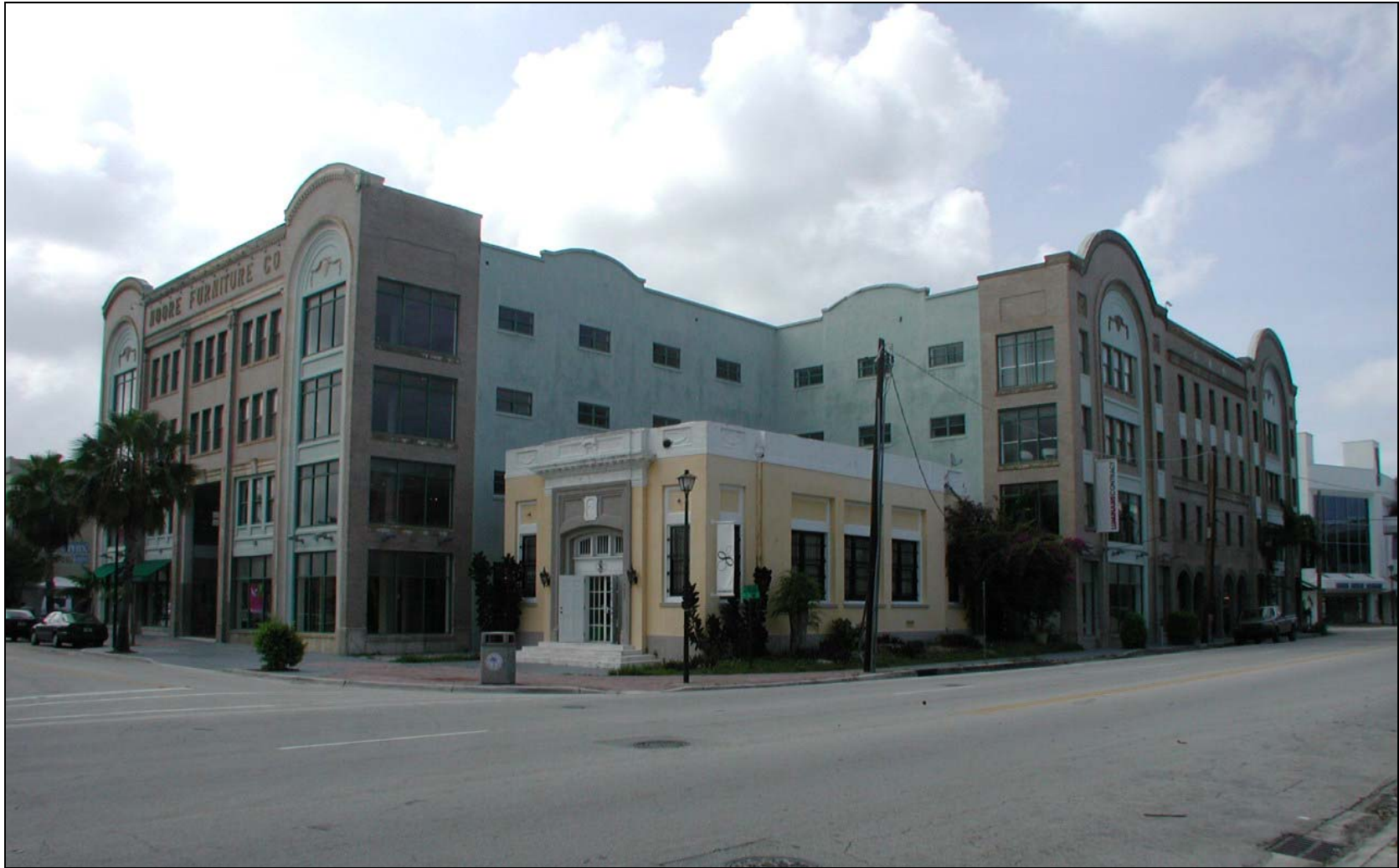
Buena Vista Post Office / Moore Furniture Building 4000-4040 NE 2 nd Avenue Photograph, facing northwest 2003
