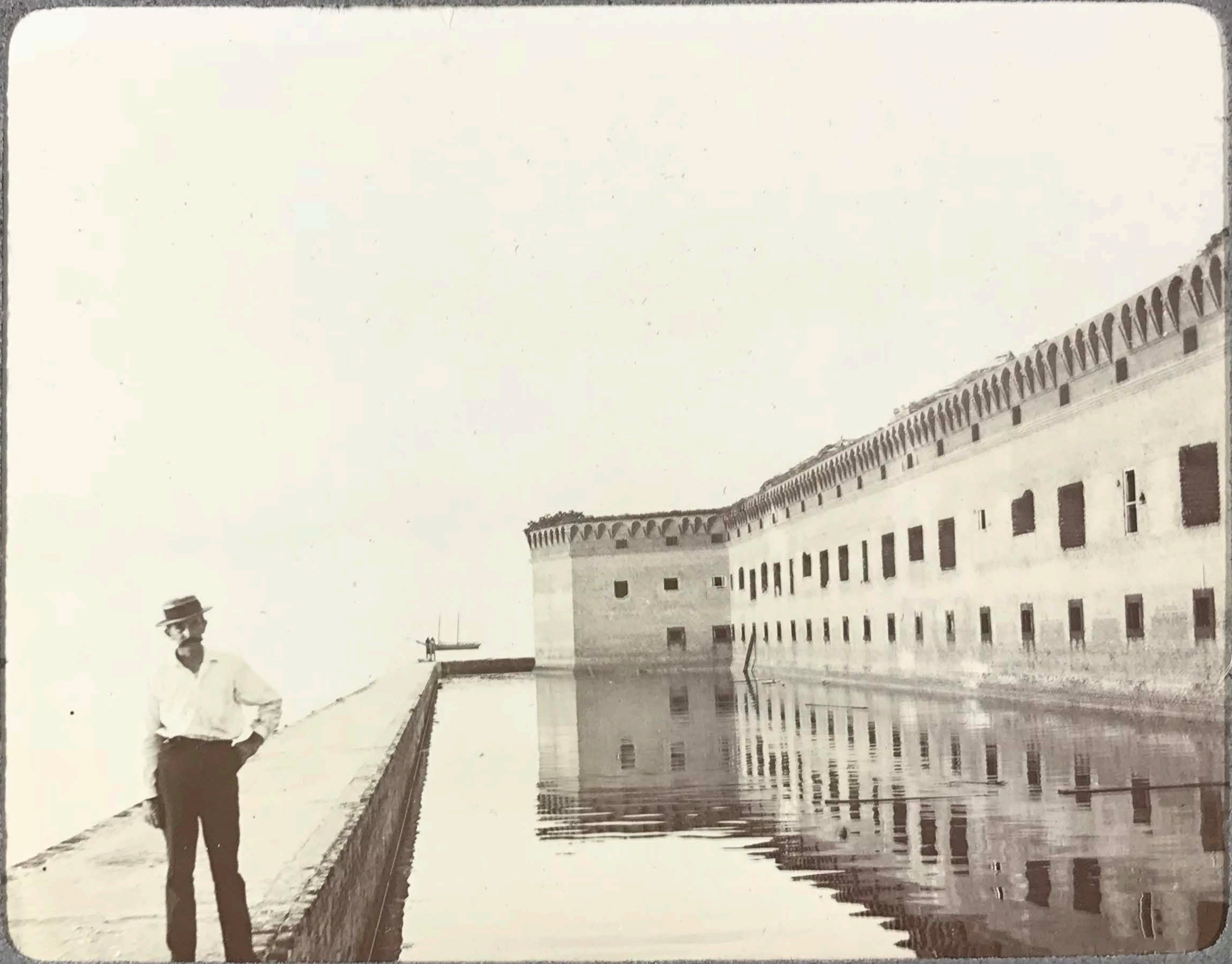
Moat, of West Face Fort Jefferson.
