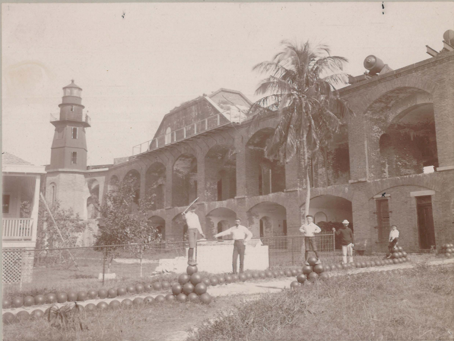
Old guard room and sally port.
