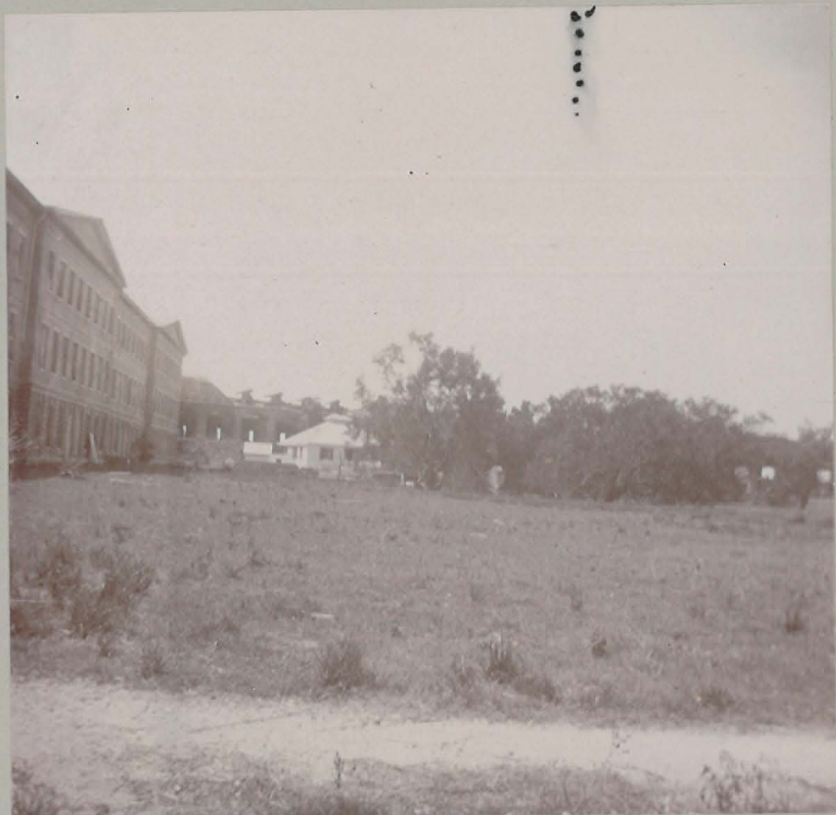
Light House Keepers Quarters.
