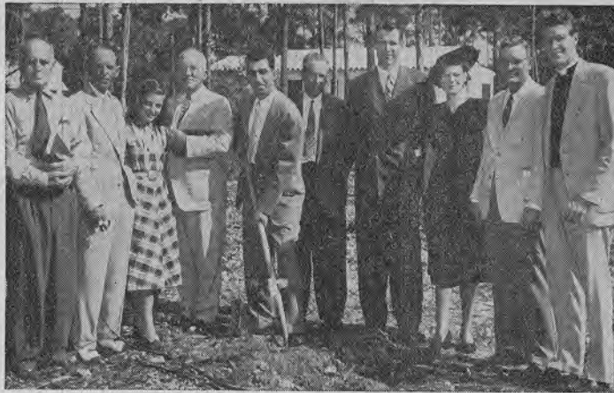
South Miami Lutherans broke ground this week for their new church edifice, construction on which is scheduled to follow. Left to right: Percy Jacobs, Clyde Shafer, Jane Shafer, E. J. Shafer, Dale Edwards, Edward Shafer, John Stauffer, Mrs. Robert Dasher, Robert Dasher and the Rev. John E. Meyer.
