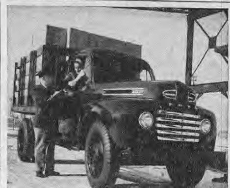
The new 1948 series F-5 Ford 1 1/2-ton, 134-inch wheelbase truck with a nine-foot stake body was shown to the public today by the Ford Motor Company. The new truck line represents the first postwar products of Ford and is offered in a wider range of models and capacities than ever before, from 1 1/2-ton pickup and panel models through 2 1/2- and 3-ton series F-7 and F-8, the largest trucks the company has ever built.
