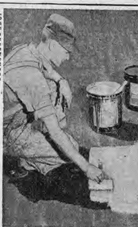
HERE'S LATEST scientific development for summertime comfort—new aluminum roof paint which forms an aluminum, foil-like, protective shield which deflects 80 percent of sun's rays and reduces interior temperatures by 15 degrees. Developed by United Gilsonite Laboratories, it is suitable for use on homes, factories and bus structures at cost of one cent a square foot. The paint also preserves roof, provides weatherproofing against sun, rain, snow, sleet, frost and dampness.
