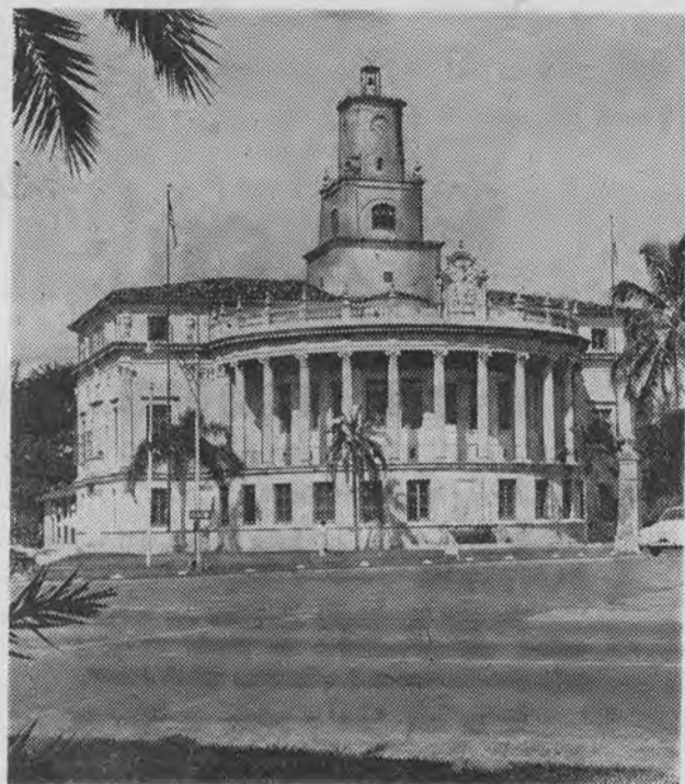
CORAL GABLES CITY HALL is one of America's most photographed landmarks, embodying design features and natural rock materials used for centuries in Europe. The coral rock structure sits at the end of the Gables' famed Miracle Mile and is at the hub of the city's downtown business district.
