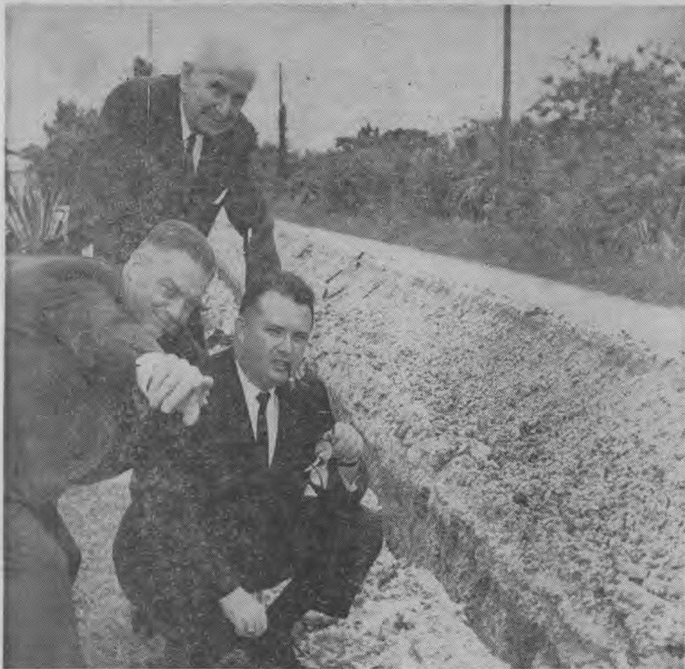
POINTING OUT where Florida Gas Co. will lay its pipeline bringing natural gas to South Miami is Owen Bowser, the firm's division manager. With him are, kneeling, City Manager Richard Barton and Mayor Paul Tevis. South Miamians
