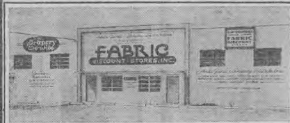
"FABRIC DISCOUNT STORES" Our Giant Modern Factory, Warehouse Offices, And Showrooms At 6950 N.W. 37th Ave.
