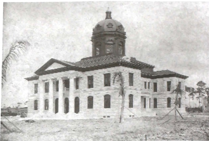
Dade County Courthouse shortly after it was constructed in 1904. HistoryMiami, x-0665-1.
