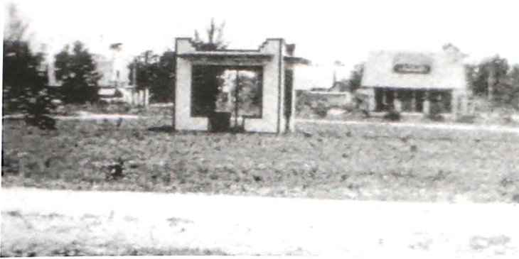
View of the park in Highland Park, looking south from NW Thirteenth Street. At the park, NW Thirteenth Street divides into north and south sections, joining again beyond the park. The shelter at the center of the park is gone, but the park itself and the house behind it (808 NW Thirteenth Street) still exist. HASF 1989-22-327.
