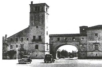
Paist and Fink also collaborated with Walter De Garmo in the design of La Puerta del Sol (Douglas Entrance), 1924-1927. Courtesy of the City of Coral Gables Historical Preservation Division.
