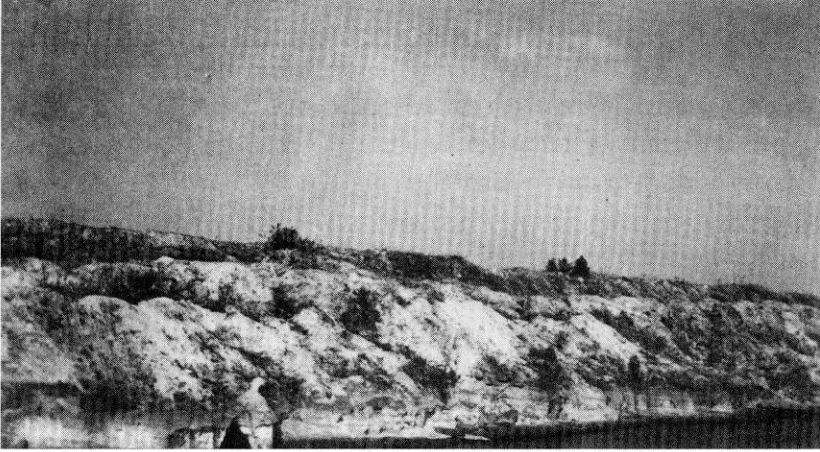
View of the high banks of Fox's Cut in Flagler County, 1915. The Florida canal company dredged this and other 'dry' cuts between the Matanzas and Halifax rivers for thirty years, off and on, from 1882 until 1912. Courtesy of the Florida State Archives.
