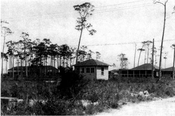
Army base buildings at the time of the site inspection by Dr. David Fairchild in 1922. View to north of hospital showing (left to right) officers' mess, quartermaster's storeroom, and officers' quarters. Courtesy of the U.S. Department of Agriculture & the archives of the Subtropical Horticulture Research Station, Miami, FL.
