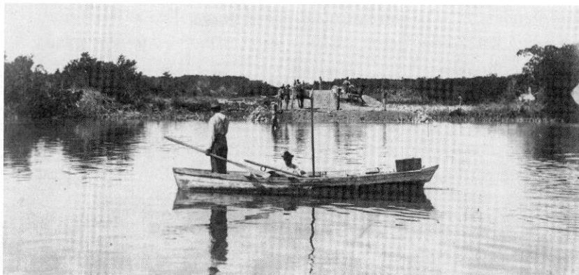
Setting stakes at Crawl Key. HASF 1991-208-34.
