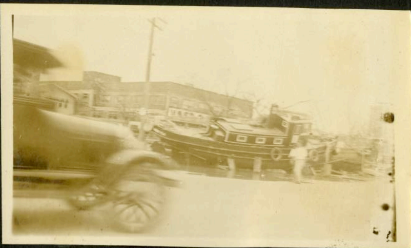
BAYSIDE DRIVE AT 11 TH ST. -
