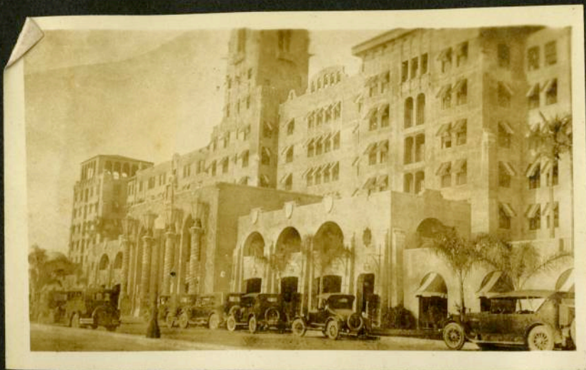
HOLLYWOOD HOTEL BEFORE - Hurricane
