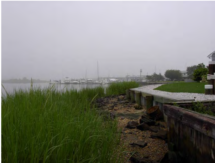
Photo 3.2: Fringing March and Bulkhead, Monmouth County, New Jersey
