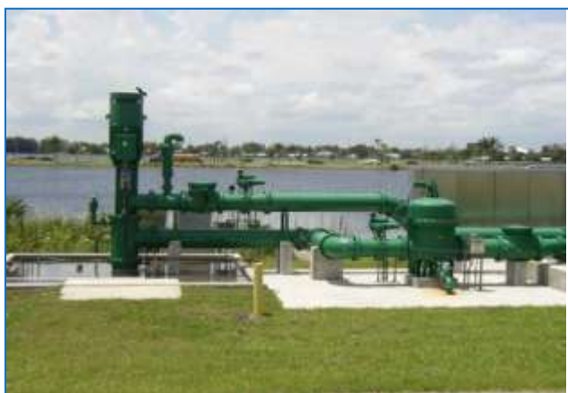
Figure 59 - A typical ASR well head.
