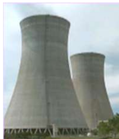
Figure 64 - Use of reclaimed water for cooling two 1 gigawatt plants in Miami-Dade County can use a total of 70-90 MGD of cooling water.
