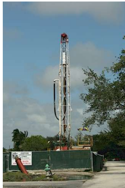
Figure 52 - Water well drilling rig
