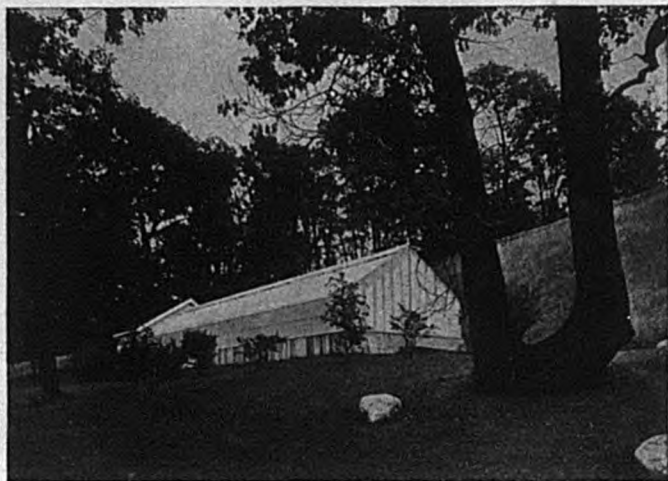
Glass Enclosed Swimming Pool
