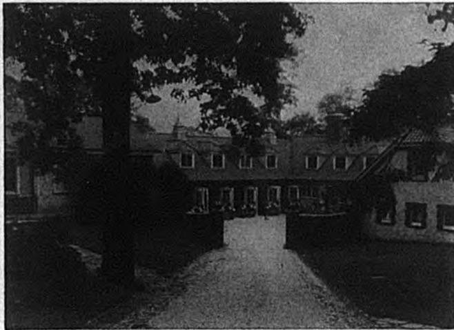
Garage and Service Quarters
