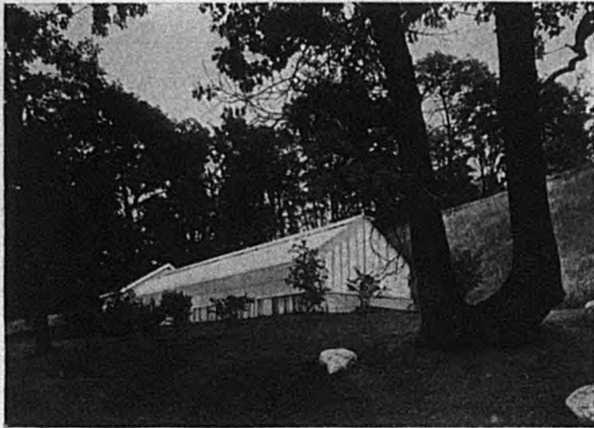
Glass Enclosed Swimming Pool
