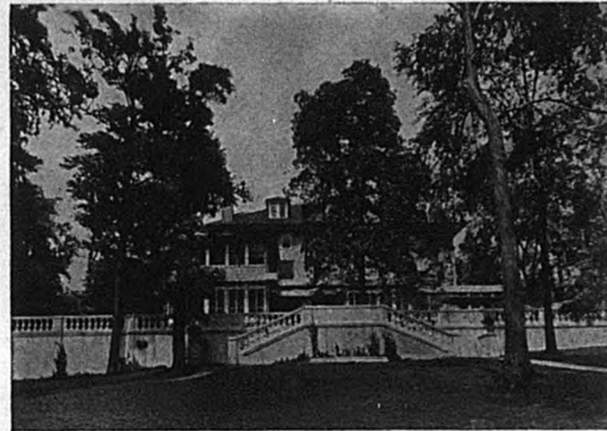
View Main House from Sound
