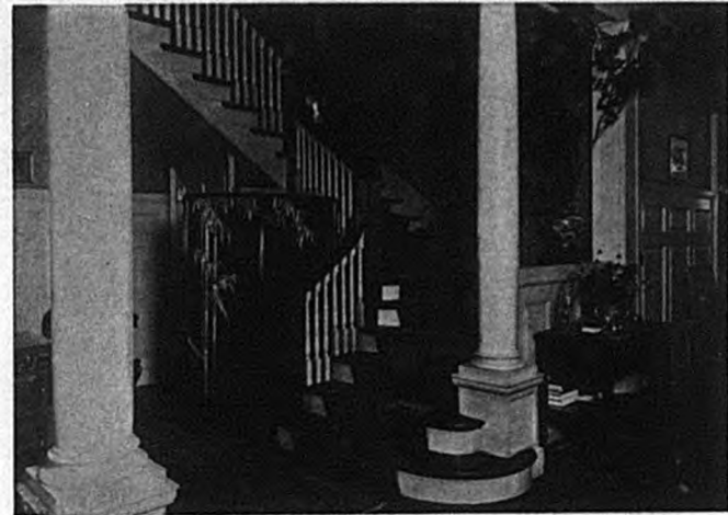
Main House Stairway
