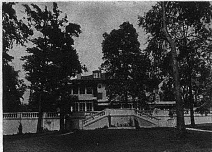
View Main House from Sound
