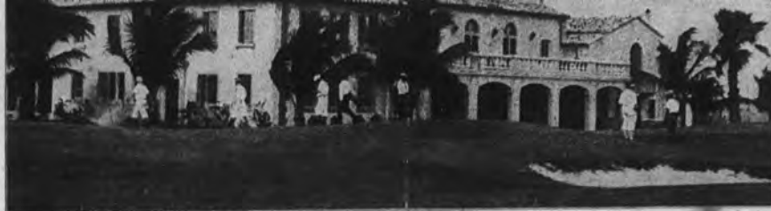
LA GORCE GOLF CLUB HOUSE, ALTON ROAD at 56th STREET
