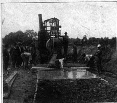
A CONCRETE ROAD UNDER CONSTRUCTION
