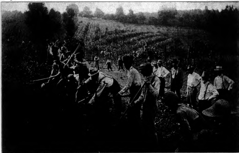
Four hundred residents of Rockcastle and Madison Counties joined forces in a road bee and worked the "Scaffold Cane" road to prove their determination to provide their portion of the Dixie Highway. Judge G. M. Ballard (with cross on sleeve), Berea students and a host of others participated in the celebration. At noon a big basket dinner was served by the women of the two counties
