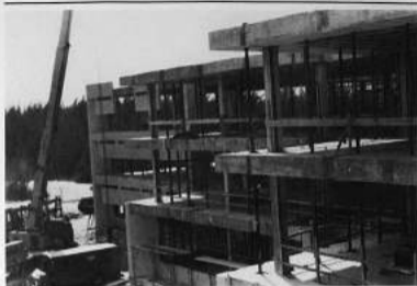
No, this is not a former airplane. It's the skeleton of Academic II which will soon include BHS's new high school as well as the art and science
