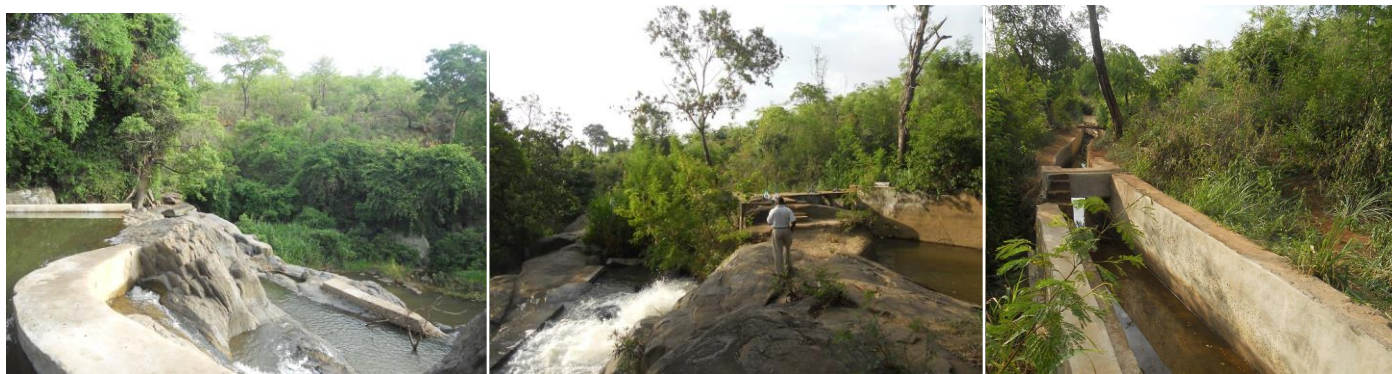
Figure 26: The Mkindo River irrigation intake
