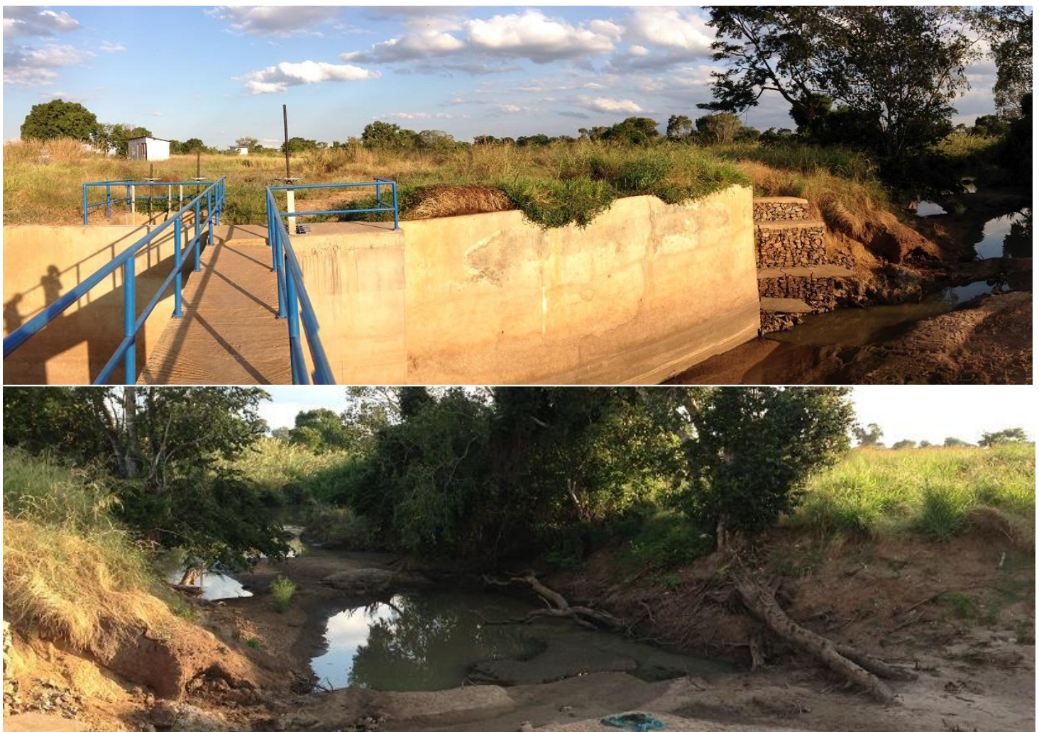
Figure 28: (Top) Irrigation intake at Lukenge, where water level marks can be painted on the wall for monitoring water level (Bottom) The Mkindo River in the dry season at Lukenge. The river rises 4 m higher in the wet season as evident from the incised channel and from local anecdotes
