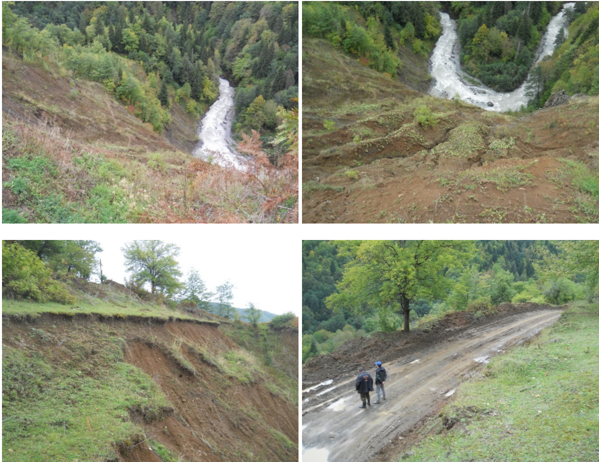
Pic. 15, 16, 17, 18. Landslide process at Sakao-Mazhieti motor road
