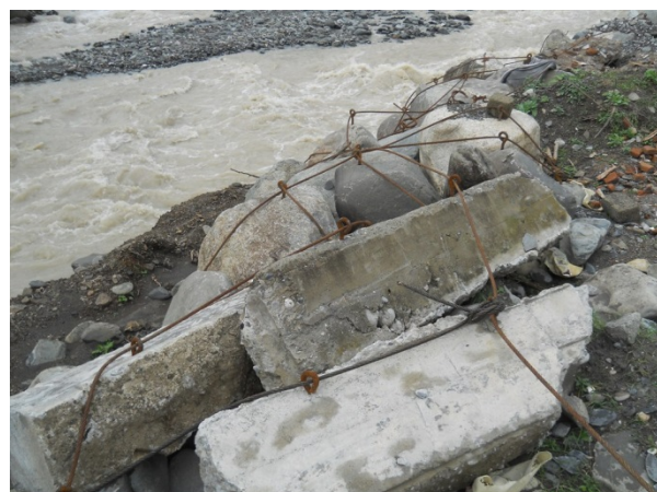
Pic. 3. The village Lagvanta. The Sakaura River. Boulders tied with wire
