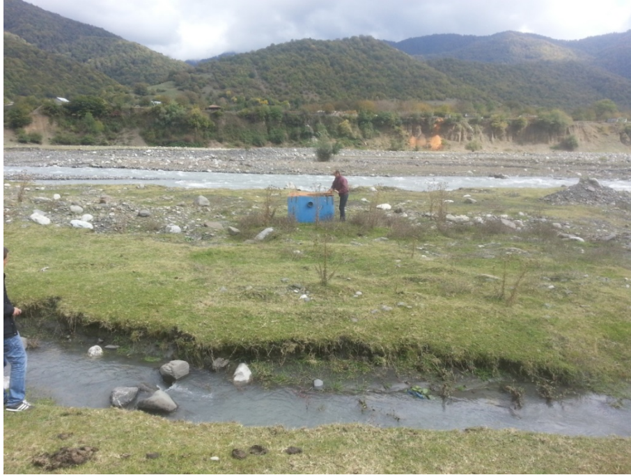
Pic. 5. The village Birkiani, location of the water distribution well in the right floodplain of the river
