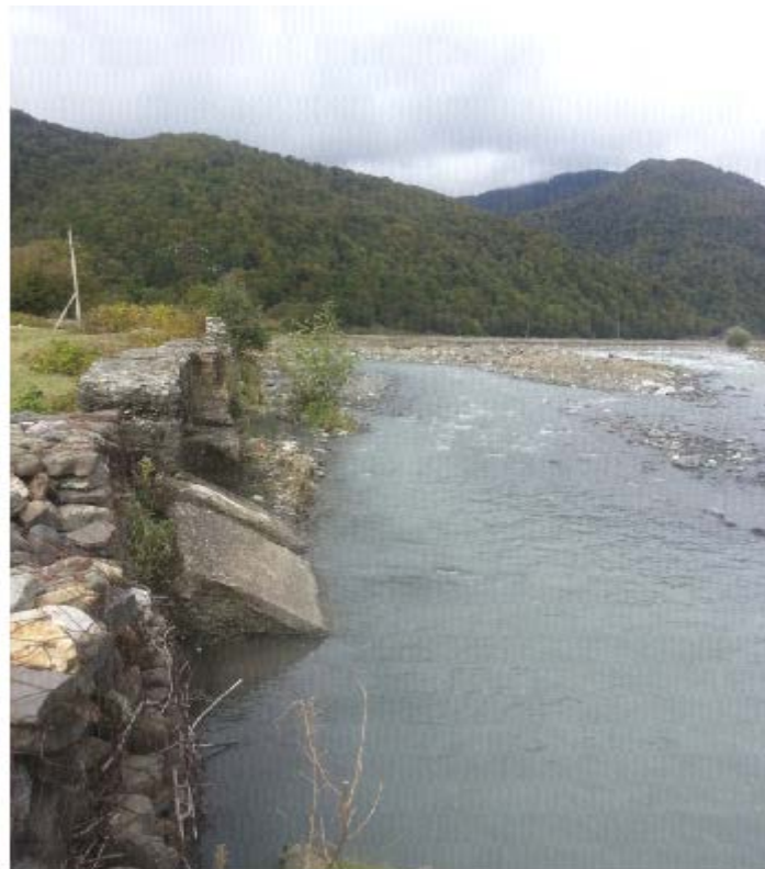
Pic. 2 The village Birkiani, the existing bank protection structure
