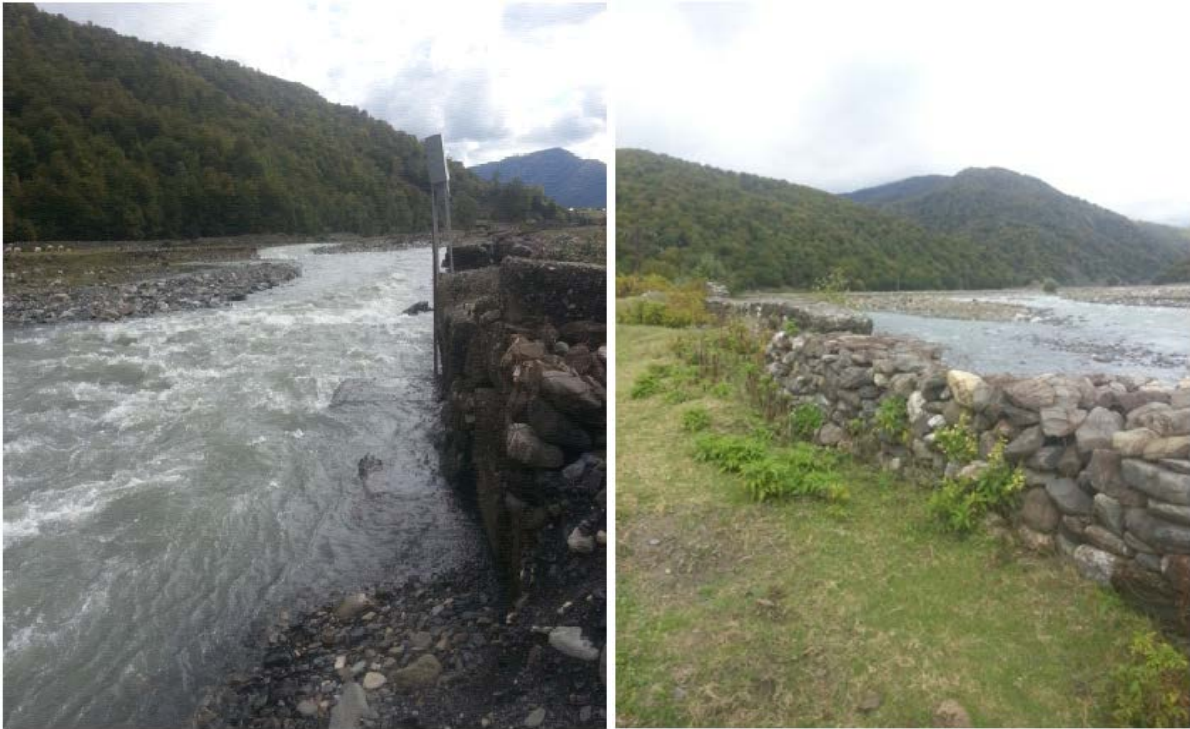
Pic. 3, 4 The village Birkiani, damped bank protection structure, protection structures of concrete and gabion type
