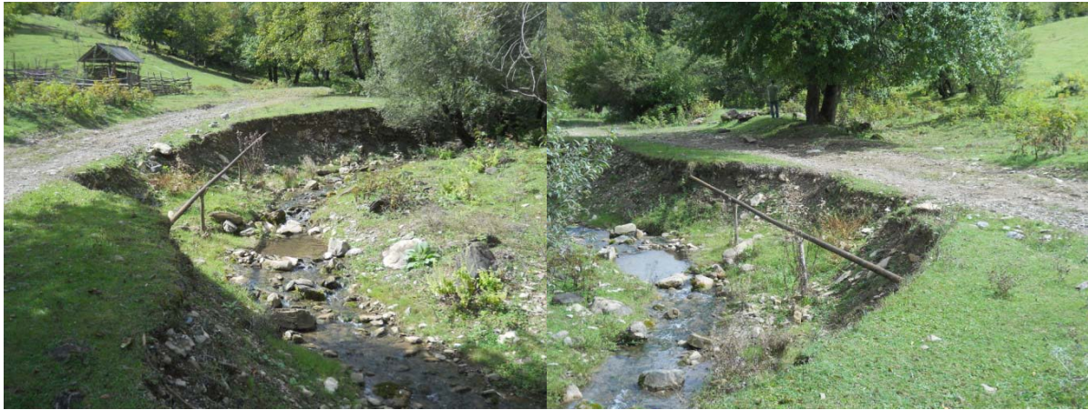
Pic. 17, 18. Erosion process occurring on the Dzibatkhevi River / bank scouring – damaged motor road
