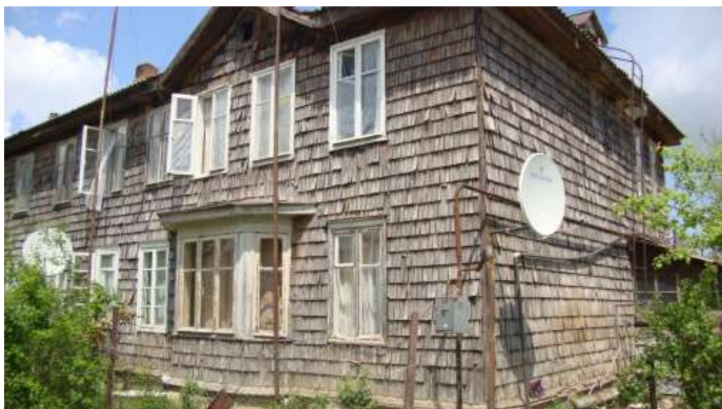
Figure 4.1 A rather unusual uninsulated house (Dedoplistskaro town)
