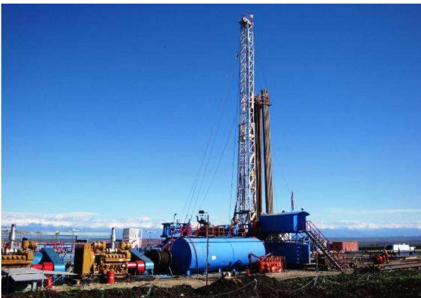
Figure 2.3 Drilling and logging operations at the Mirzaani #1 well in November 2009
