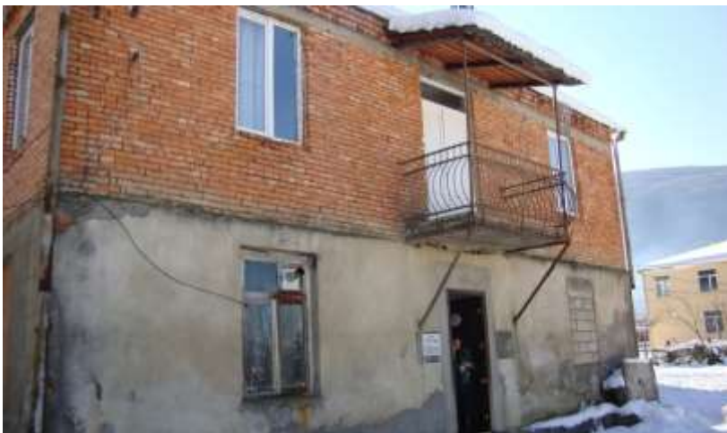
Figure 4.6: Energo Pro Company Branch Office in Ambrolauri. The facility is also heated with a wood stove.
