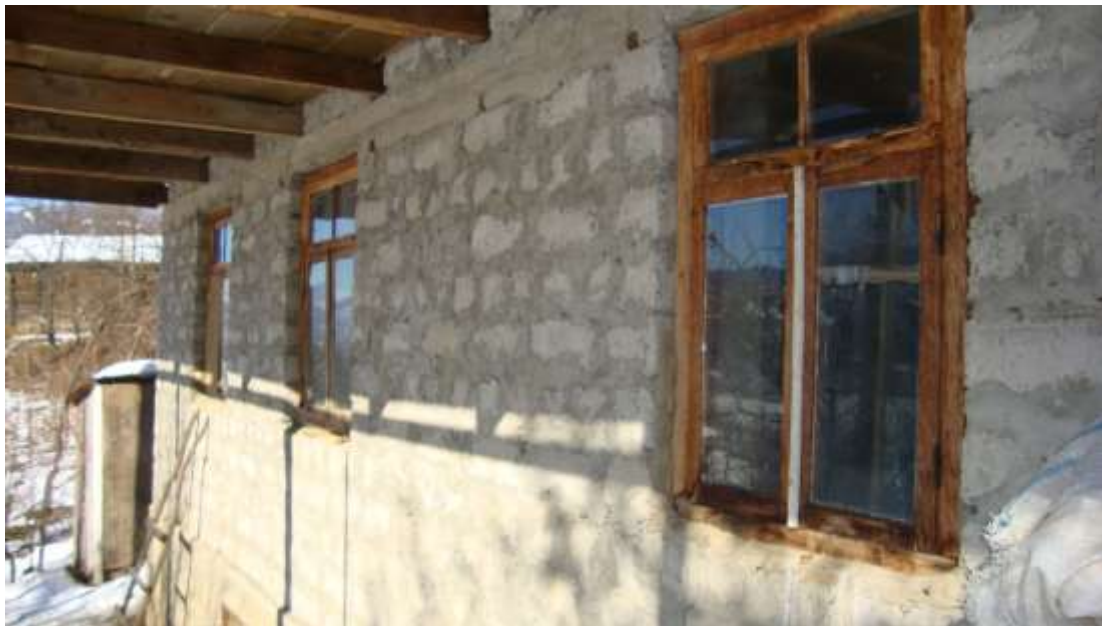
Figure 4.8: Typical Single Glazed Windows with Non-Weatherized Frames
