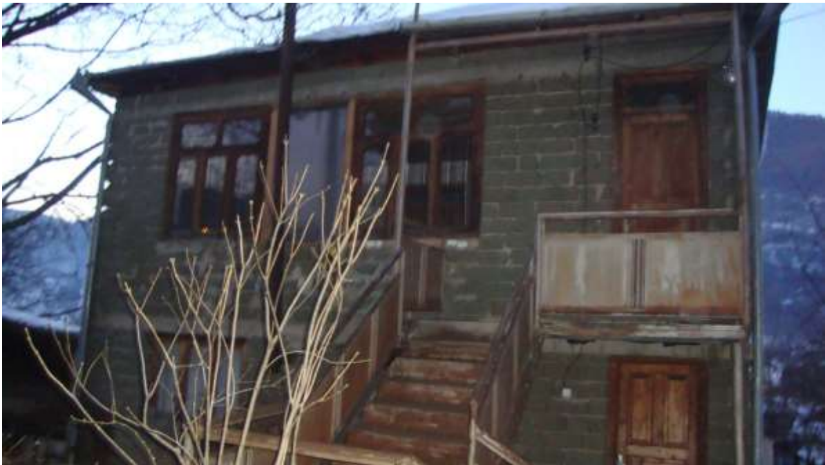
Figure 4.7: Typical Un-insulated Cement Block House with Poor Thermal Characteristics.
