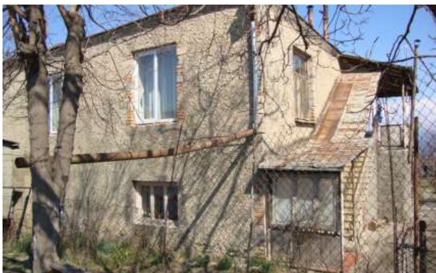
Figure 4.2: Typical uninsulated house (Ikalto village, Telavi municipality)
