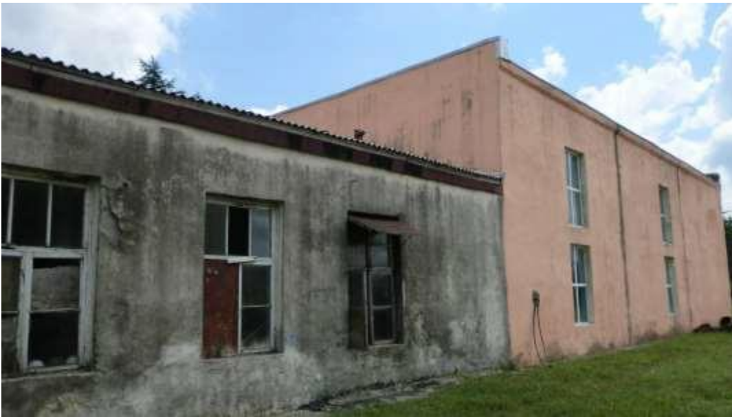
Picture 10. Rehabilitated Pumping Station and Old Premises of Operations Unit
