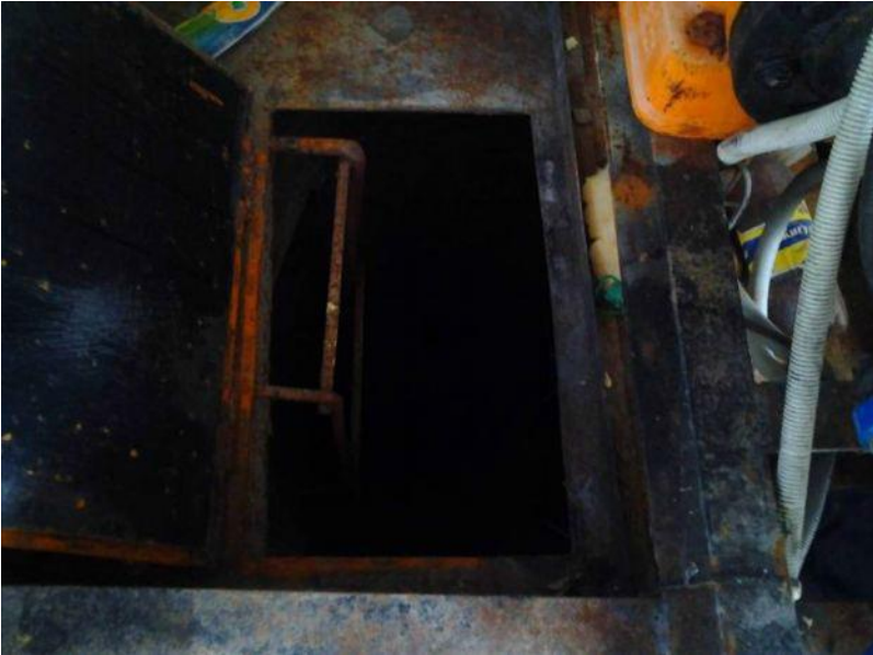
Picture 8. Shaft Well at Stadium Headworks
