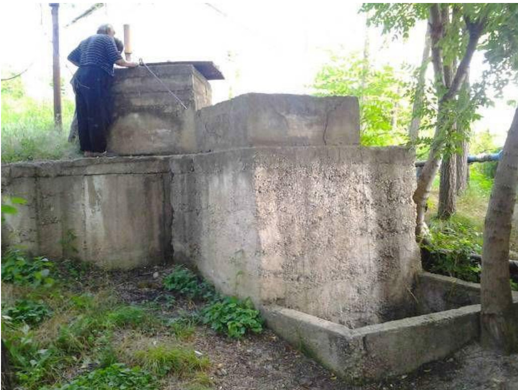
Picture 2. Mazovka Water Collection Reservoir
