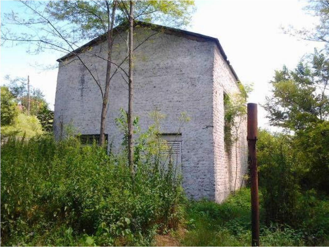
Picture 3. Former Chlorination Station at Mazovka Headworks
