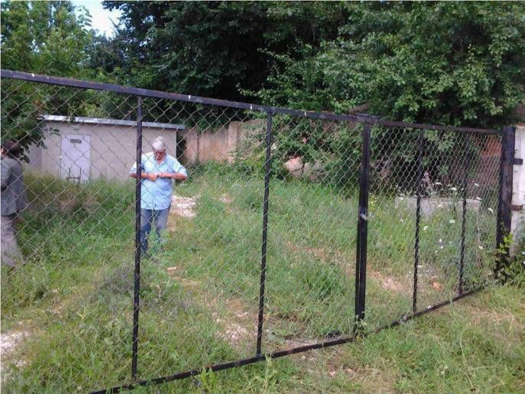
Picture 10. Sanitary Zone of the Stadium Headworks
