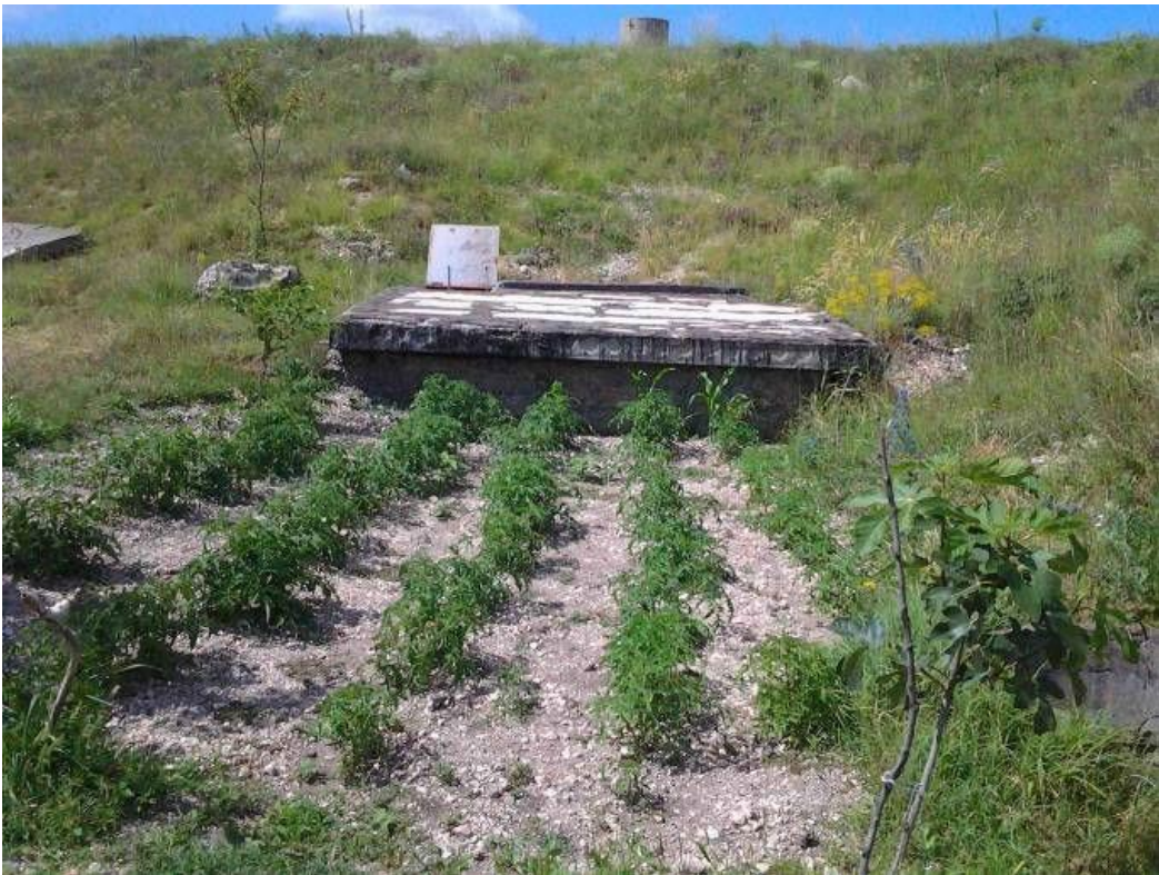
Picture 15. Regulation Unit of the Regulating Reservoir
