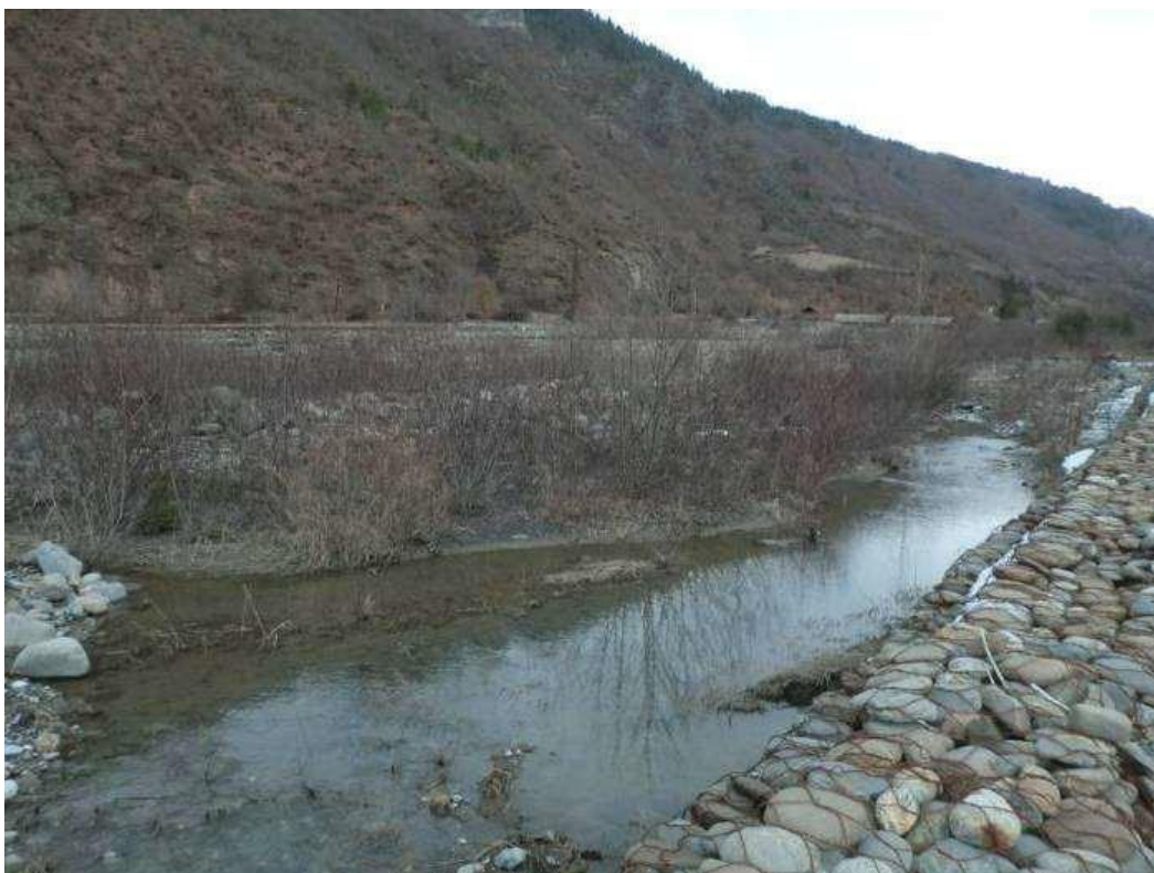
Pic. 6. Gabion at “Zhizhoreti” headworks
