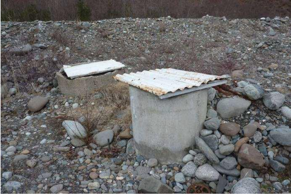
Pic. 9. Drainage well at the headworks of "Zhizhoreti"
