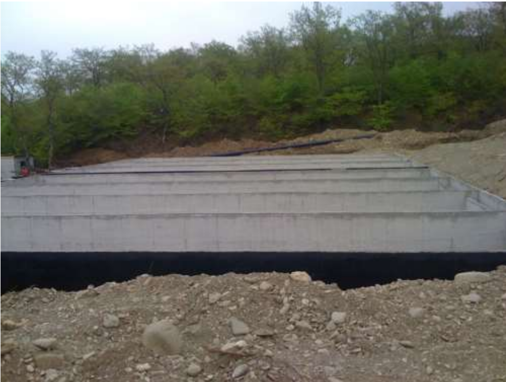
Picture 3. Constructing horizontal settler
