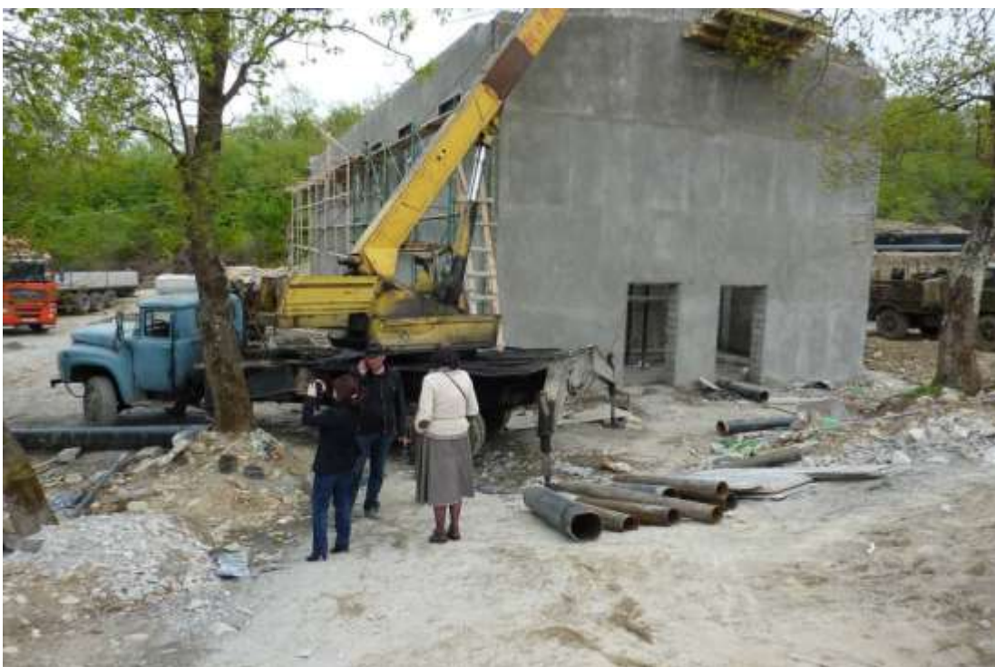
Picture 2. Constructing new drinking water treatment plant
