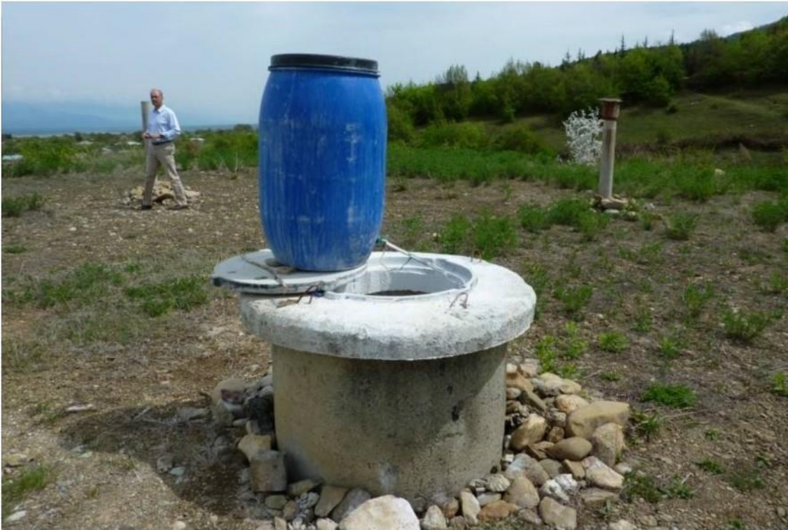
Picture 3.1 and 3.2. Process of chlorination in #1 and #2 reservoirs
