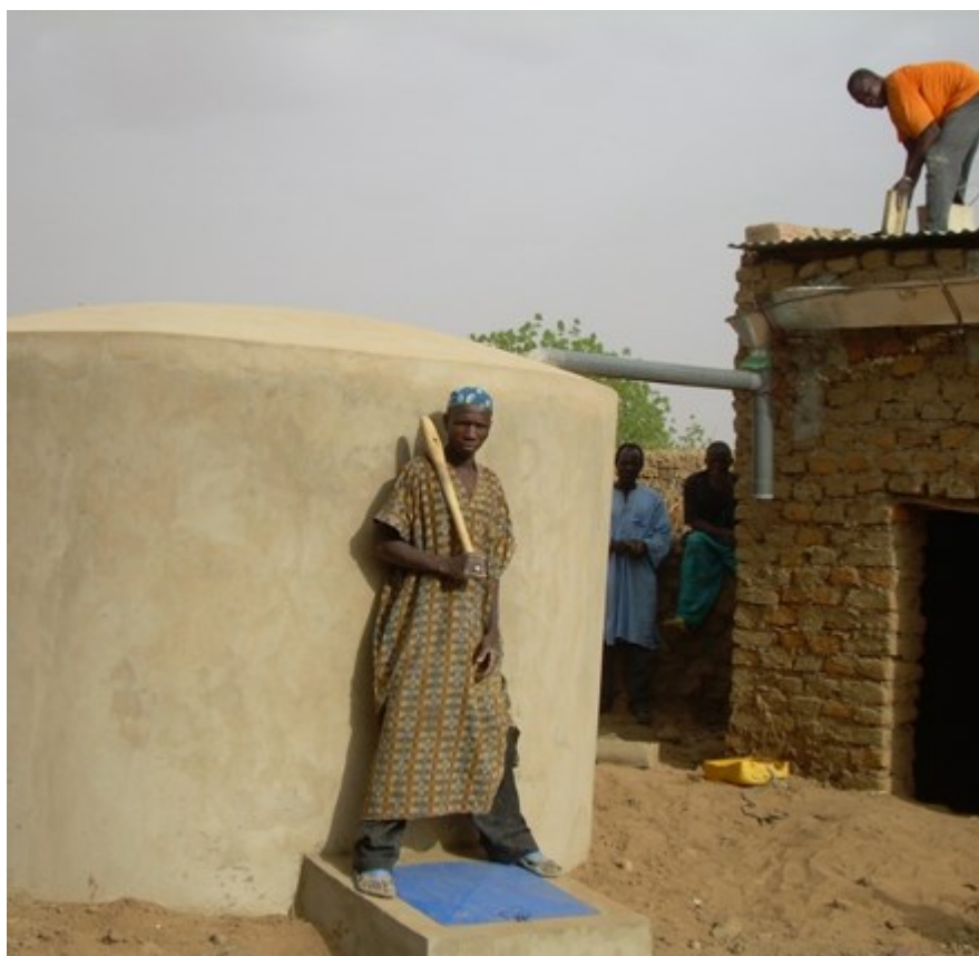
A rain water harvesting tank built in Moussoua.
