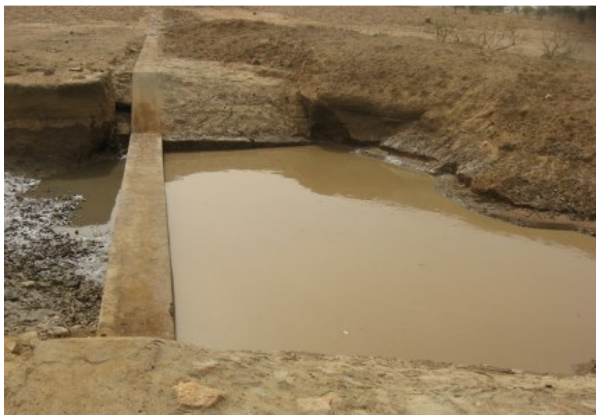
A sand dam in Tiéna holds water after an early rain.
