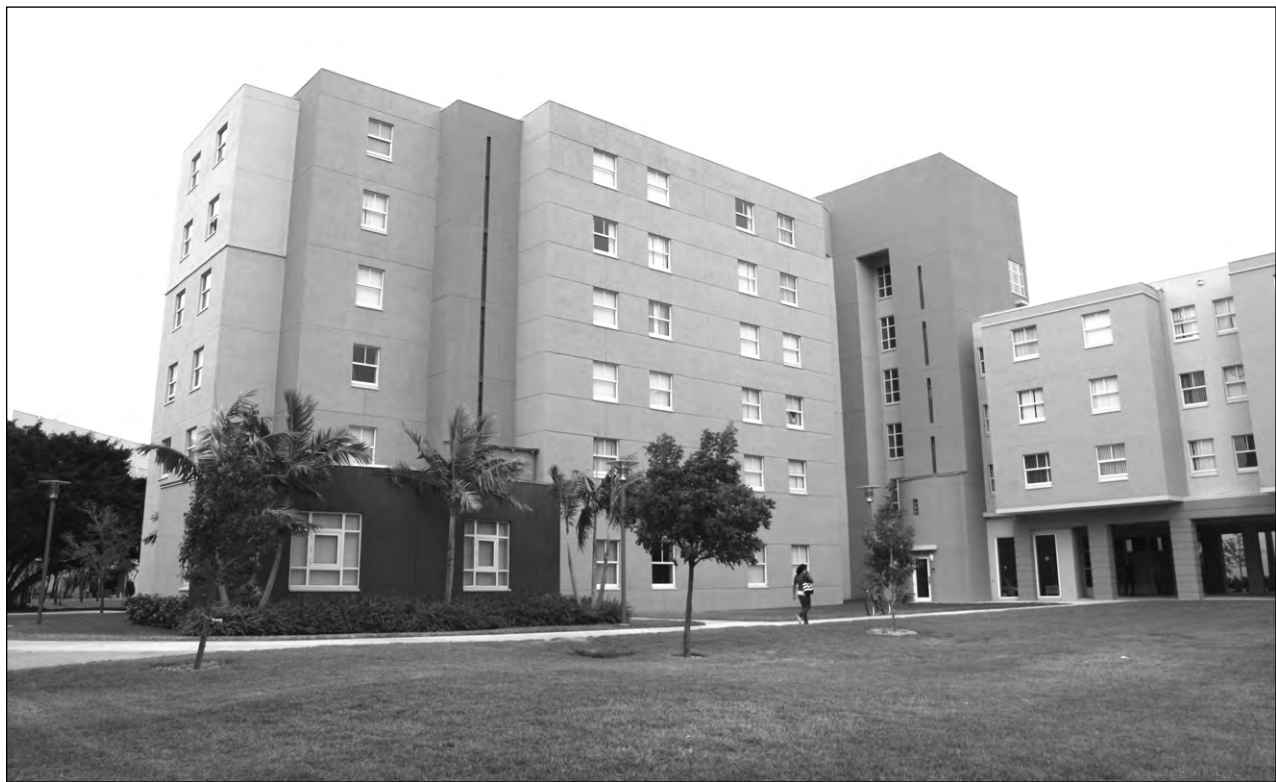
FERNANDO GARCIA/THE BEACON
