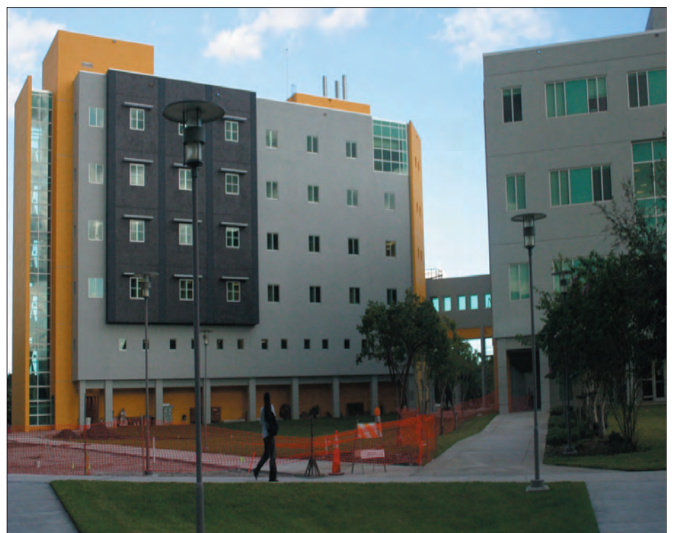
MOVIN' ON UP: The expansion of the Health and Life Sciences building is an example of FIU's readiness to open a medical school. JOHN LOVELL/THE BEACON
