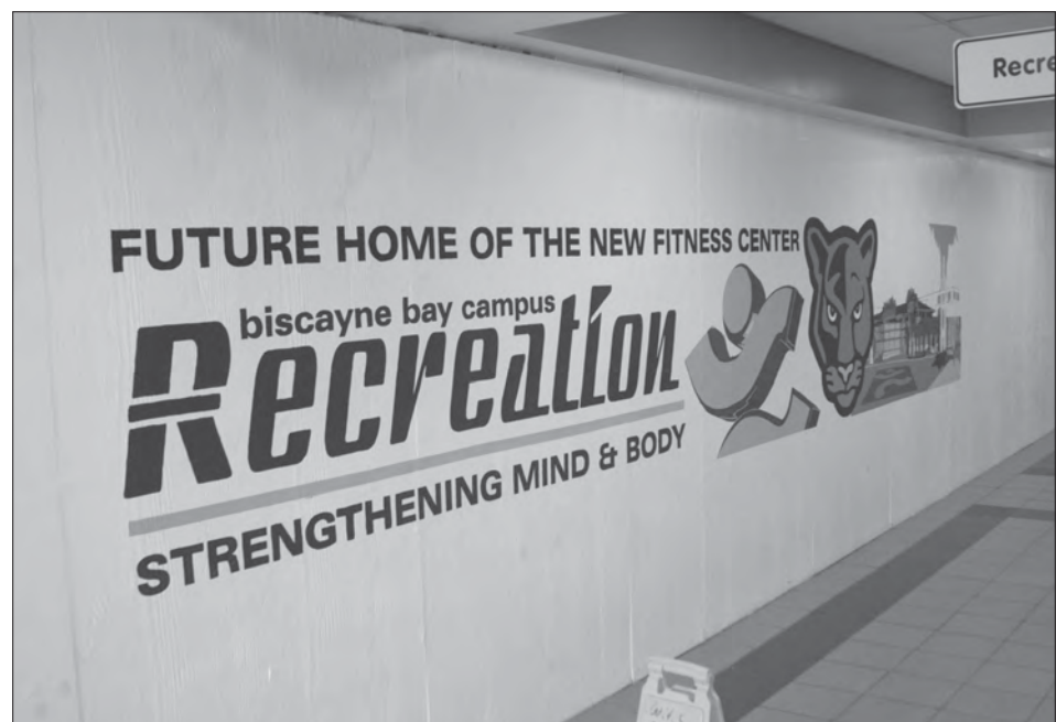
BEHIND THE WALL: Biscayne Bay Campus Fitness Center construction continues as planned and is scheduled to open in January 2006. ISIDRO PENTZKE/THE BEACON
