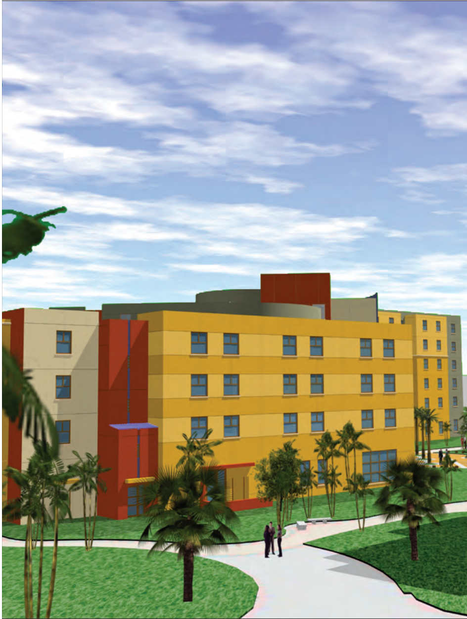
LAKEVIEW: Turner Construction has begun phase one of the new 250,000 square foot, Lakeview housing units at University Park. FIU Housing is hoping to be able to accommodate 3,000 more students with the new addition. COURTESY PHOTO
