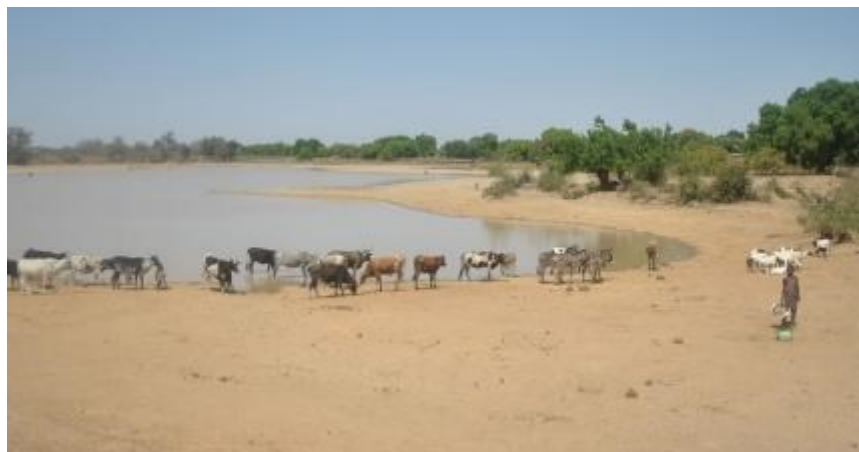
The dam in Koukouldi, the main water source for farmers and gardeners.
