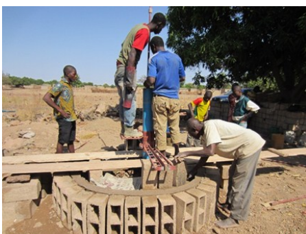
Drilling inside a due well for upgrading
