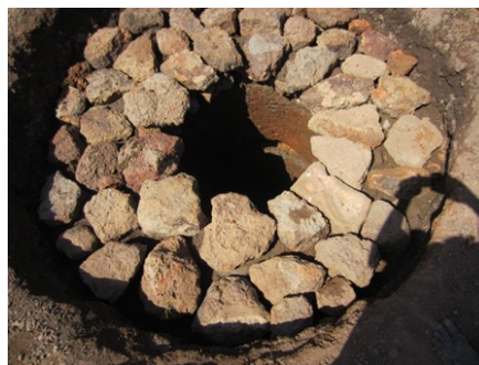
Upgrading of the top of a traditional well in Oueglega
