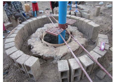
Drilling inside a due well for upgrading
