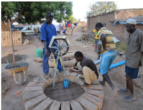
Rope pump installation in the village of Tiogo-Mossi, Burkina Faso
