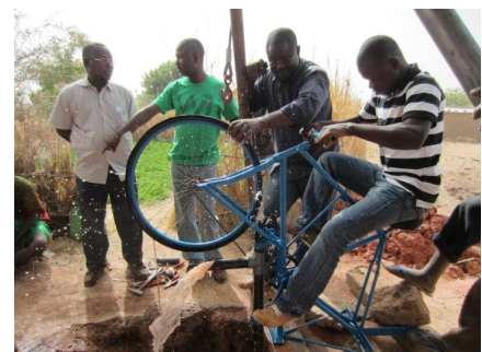
A rope pump made with a recycled bike in the village of Oueglega
