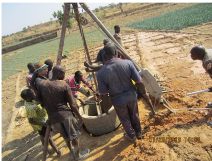
The introduction of a nozzle in a collapsed well in Koukouldi
